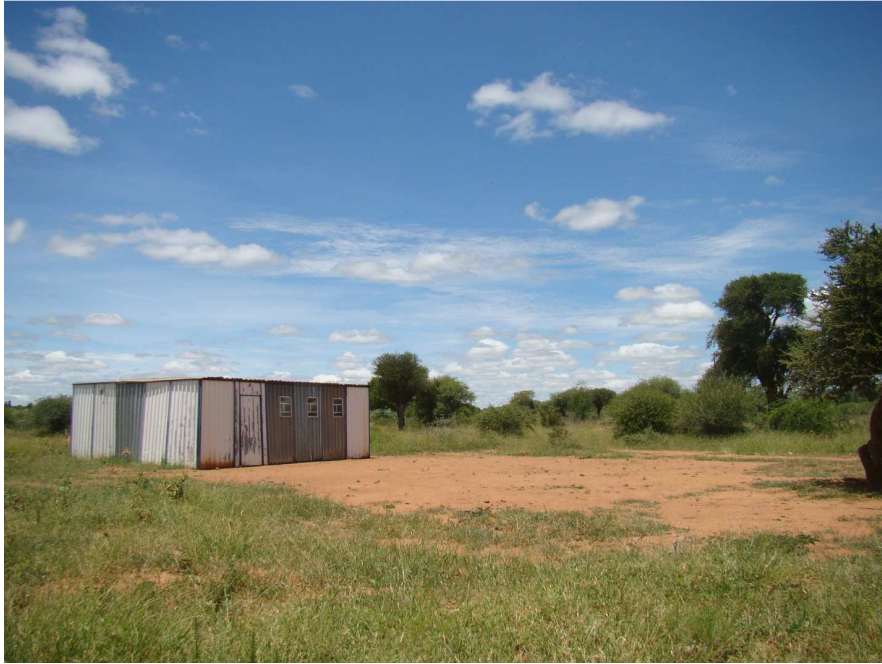
Fig. 7: The central section. Sections have been demarcated by locals with fences or corrugated iron structures for private use.
