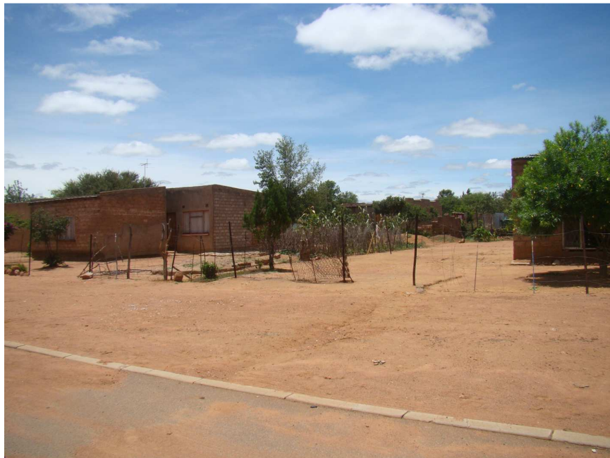
Fig. 2: Although the township is not yet formalised, infrastructure such as tarred or concrete roads, electricity and water has already been established.
