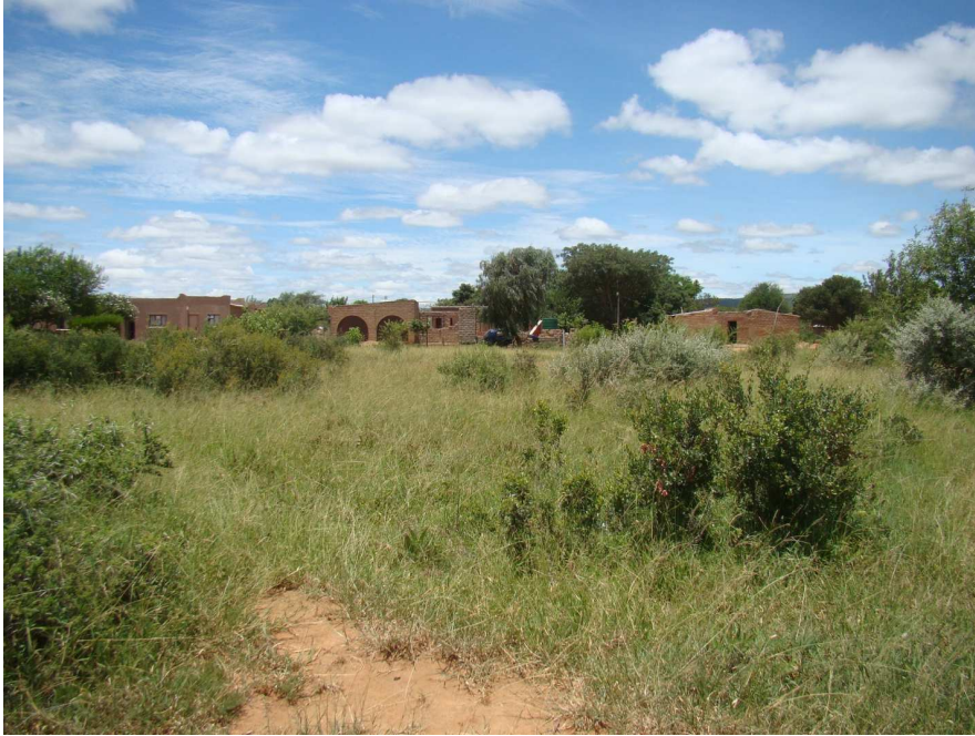
Fig. 5: View from the central / eastern section facing south. The established housing infrastructure is clearly visible. Grass and small shrubs cover most of this section.
