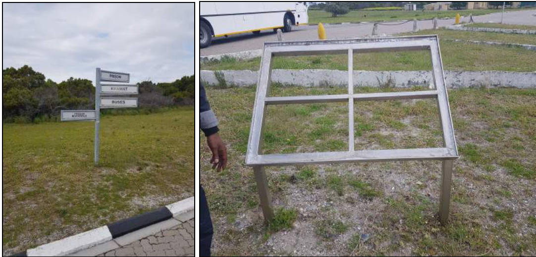
Figure 5.1 and 5.2: Prison Precinct - old signage to be replaced and made consistent
