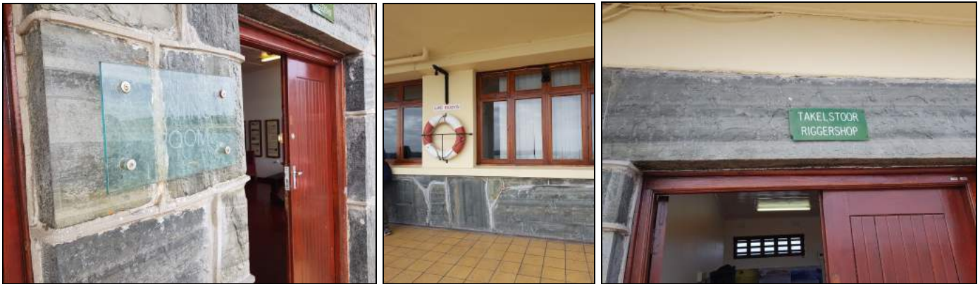
Figure 3.3, 3.4 and 3.5: Murray Harbour Office - note variable signage and artefacts eg life buoy
