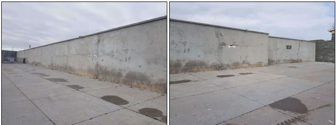
Figure 3.1 and 3.2: Murray Harbour wall
