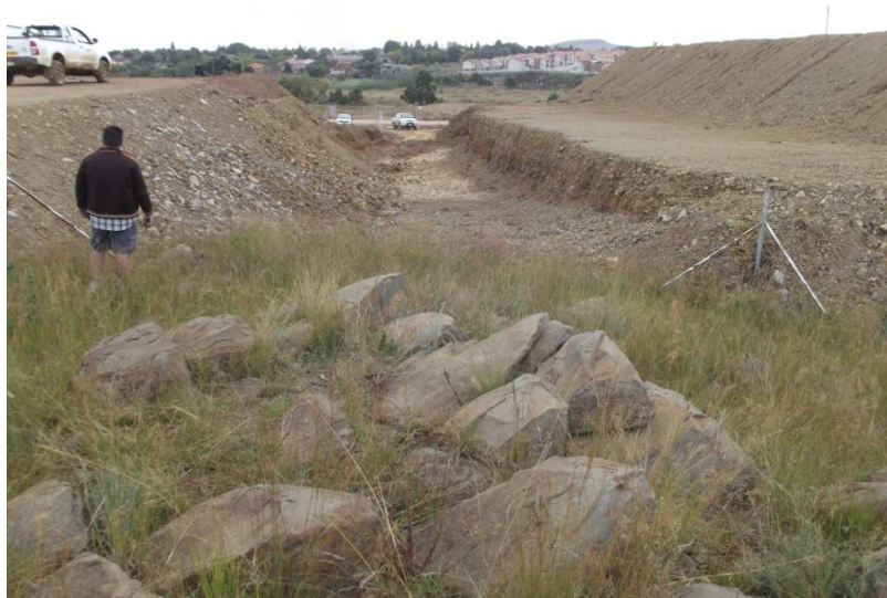
Fig. 3: Current view of the area after construction has commenced. Access was extremely difficult.
