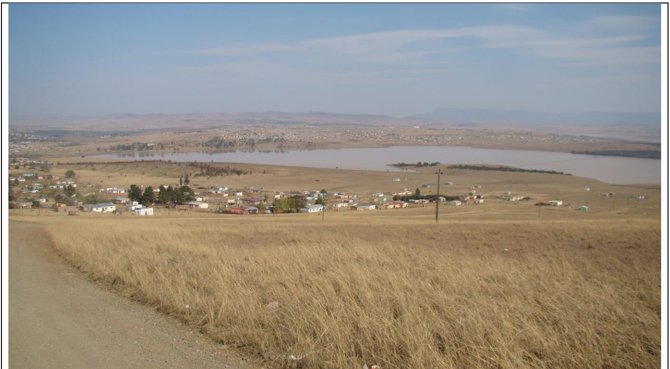
Plate 9: Photo 11 shows pipeline route along road servitude (Author 2014). Note built up sections along the proposed pipeline route
