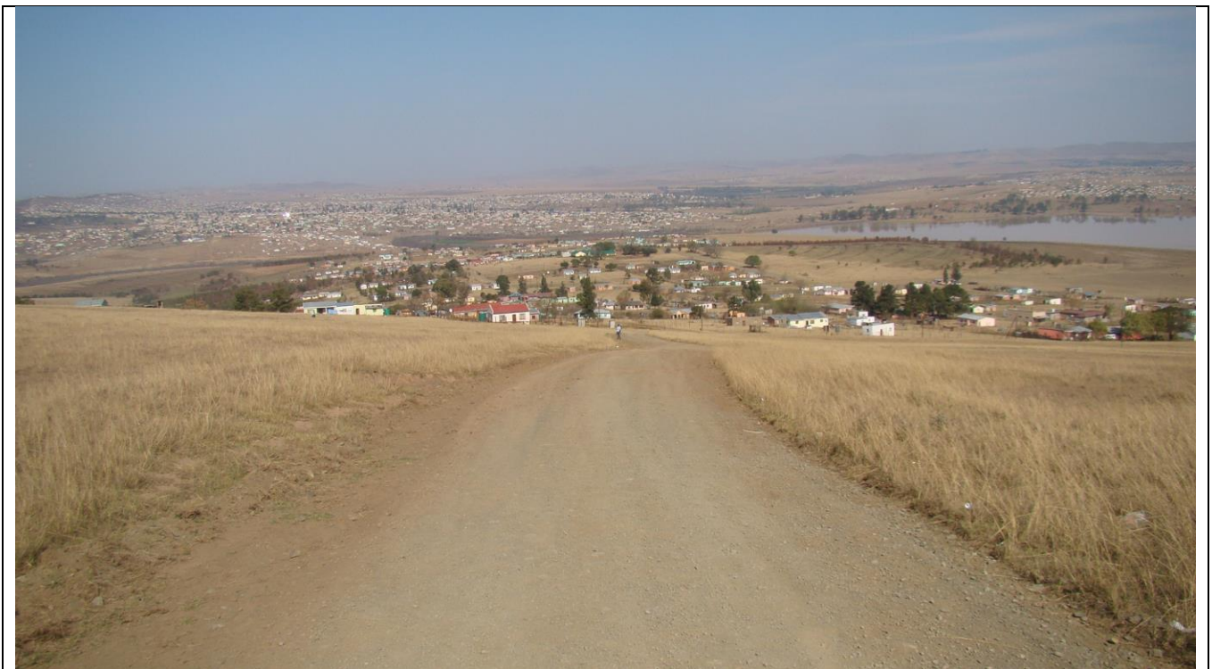
Plate 11: Photo 13 shows pipeline route along Highbury Road servitude (Author 2014).
