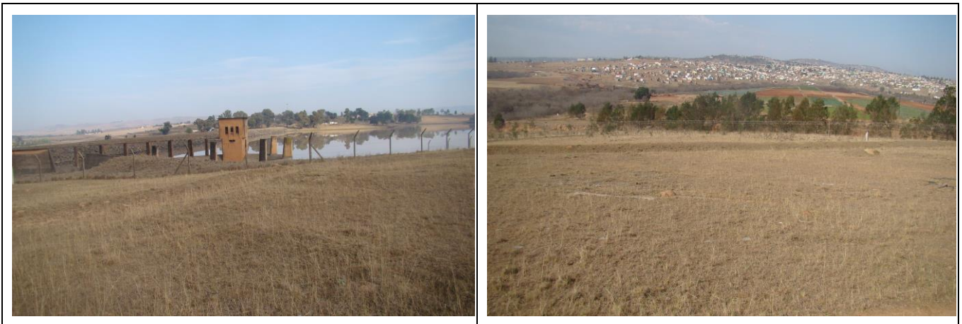
Plate 2: Photos 2 (left) and 3 (right) shows Mthatha Dam wall and section where the proposed pipeline route will cut through from the proposed pump station (Photos by Author 2014).
