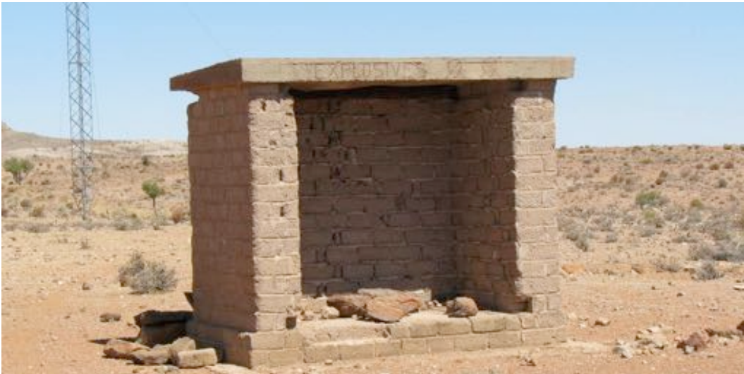
Figure 5. Remains of pre-1961 mining infrastructure.
