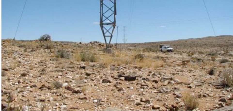
Figure 6. Minimal disturbance in the vicinity of a tower on an existing transmission line.
