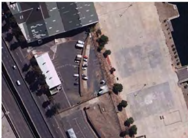
Figure 11: Existing relic of Amsterdam Battery
