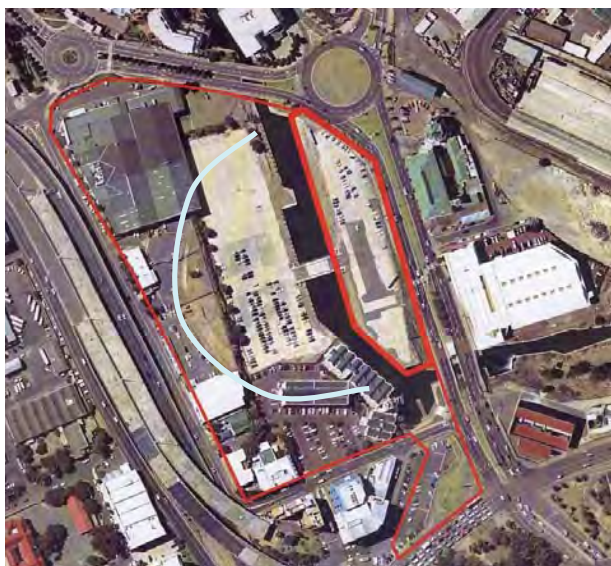
Figure 2: Detail of the Gateway Precinct showing the approximate arc of the Amsterdam Battery. The area to the north east of the archaeological remains of the Battery has been excavated to the level of the reclaimed land.
