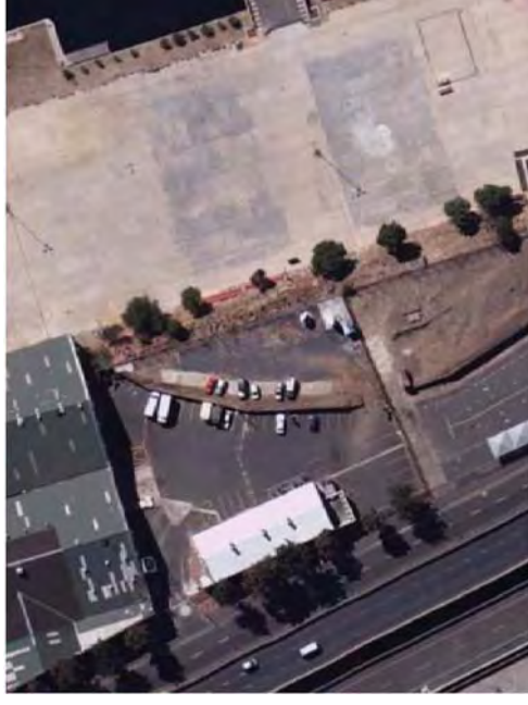
Existing relic of Amsterdam Battery
