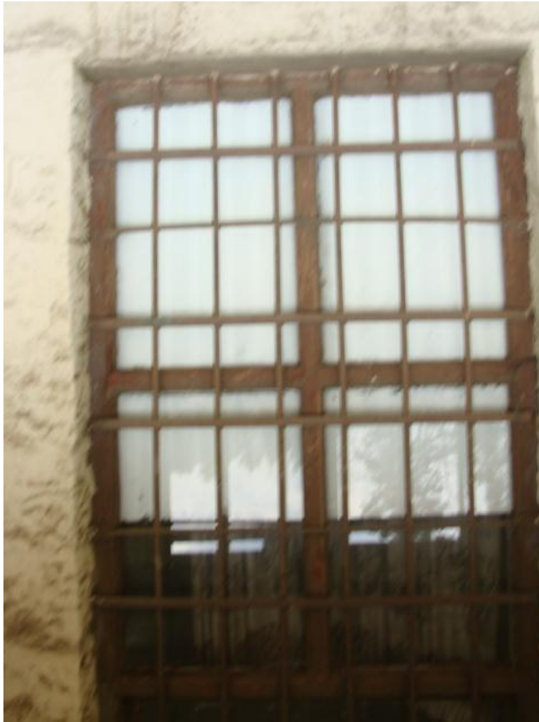
Figure 27 One of the windows in the northern façade.
