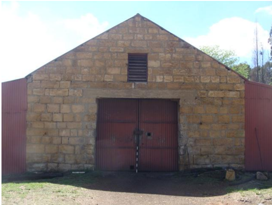
Figure 10 Detail of front façade.
