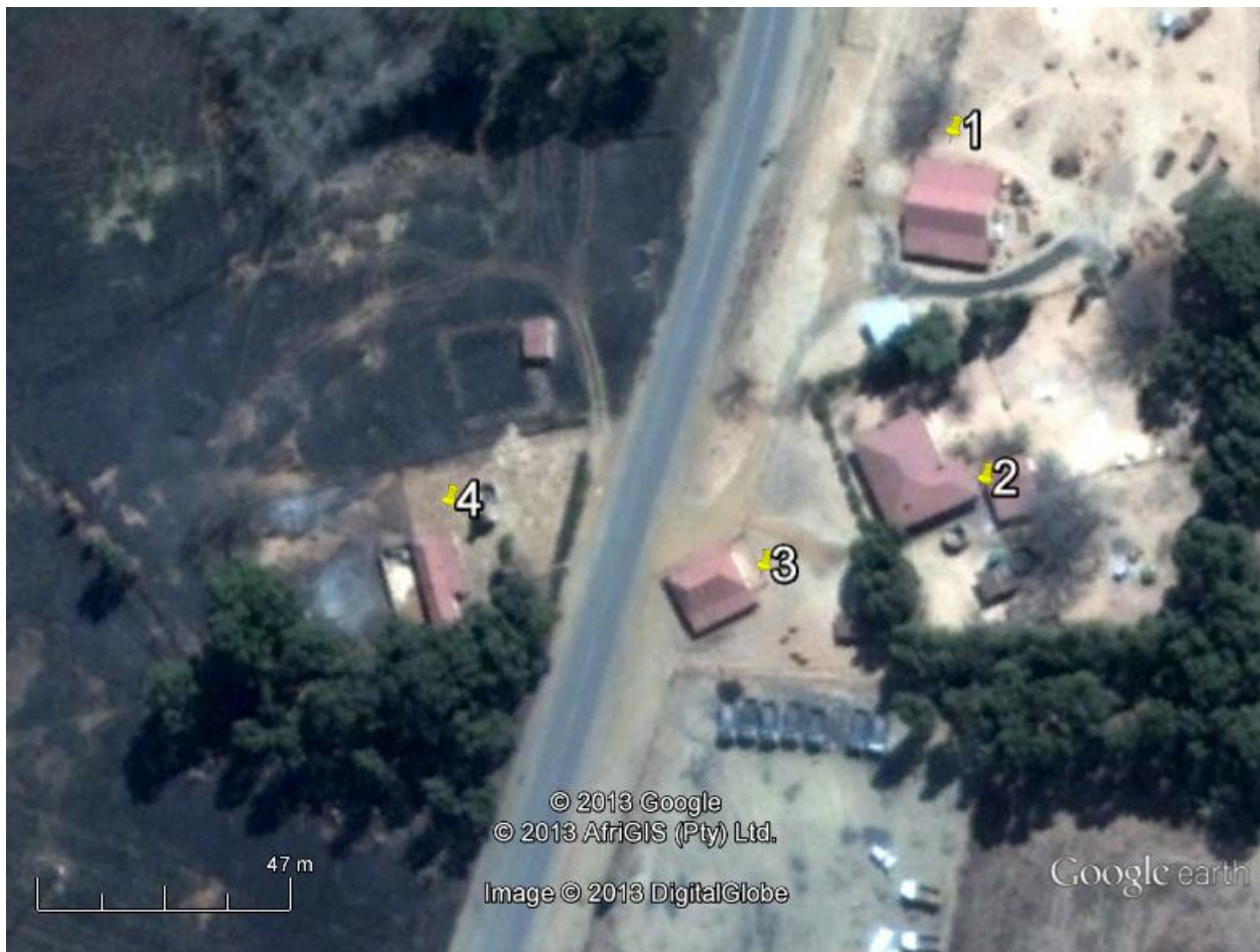
Figure 7 The farm yard indicating the four buildings discussed in this report.
