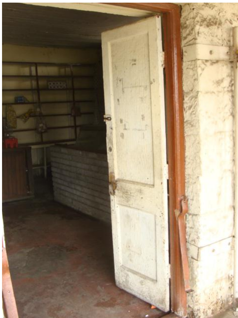
Figure 26 Door in the northern façade.
