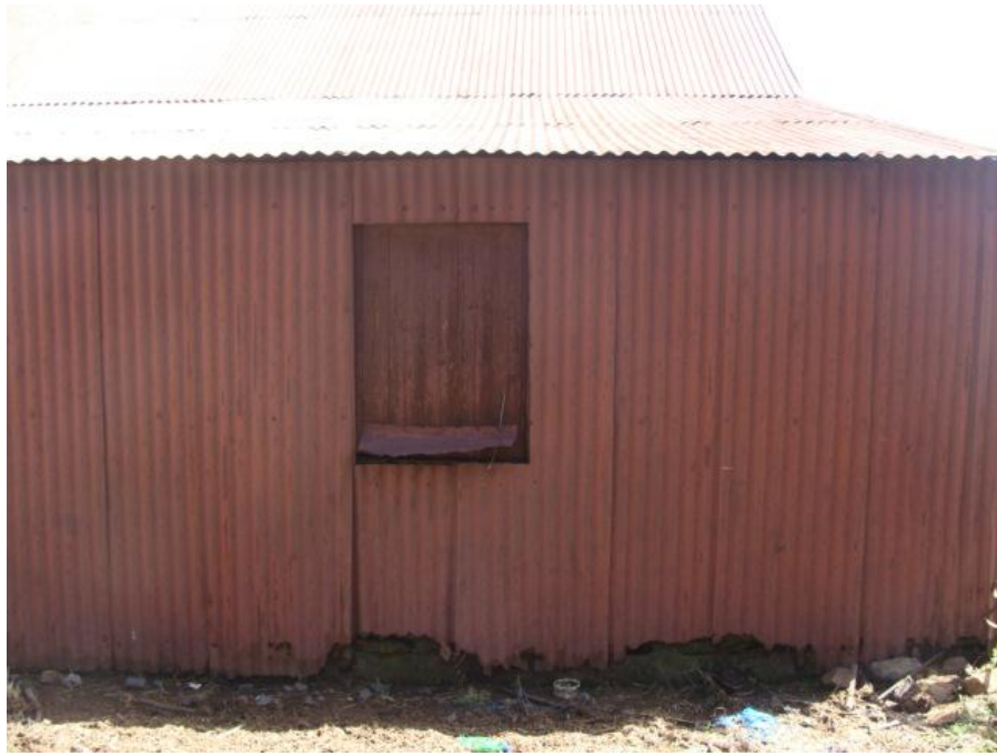
Figure 15 Detail of southern façade.
