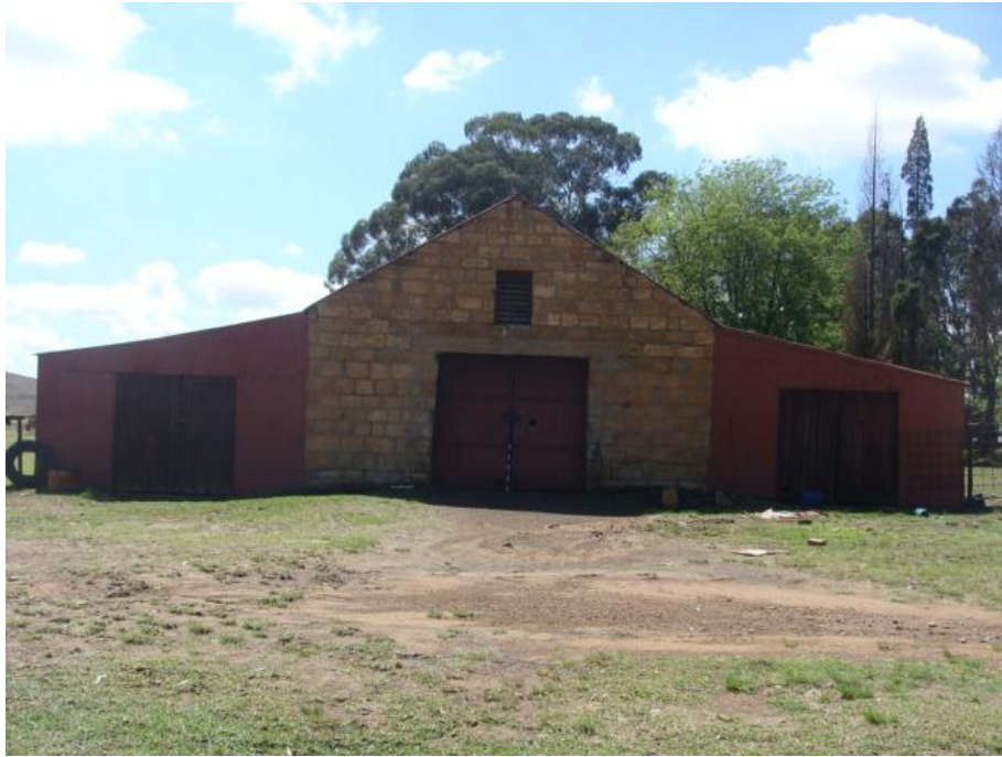
Figure 9 Front (western façade).
