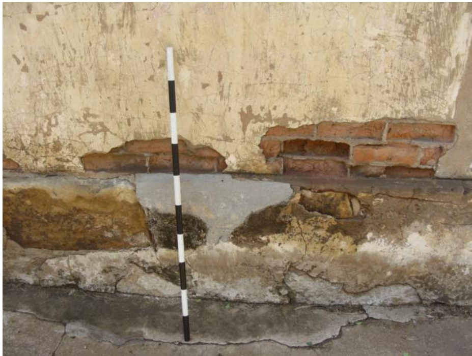
Figure 23 Foundation of the building.
