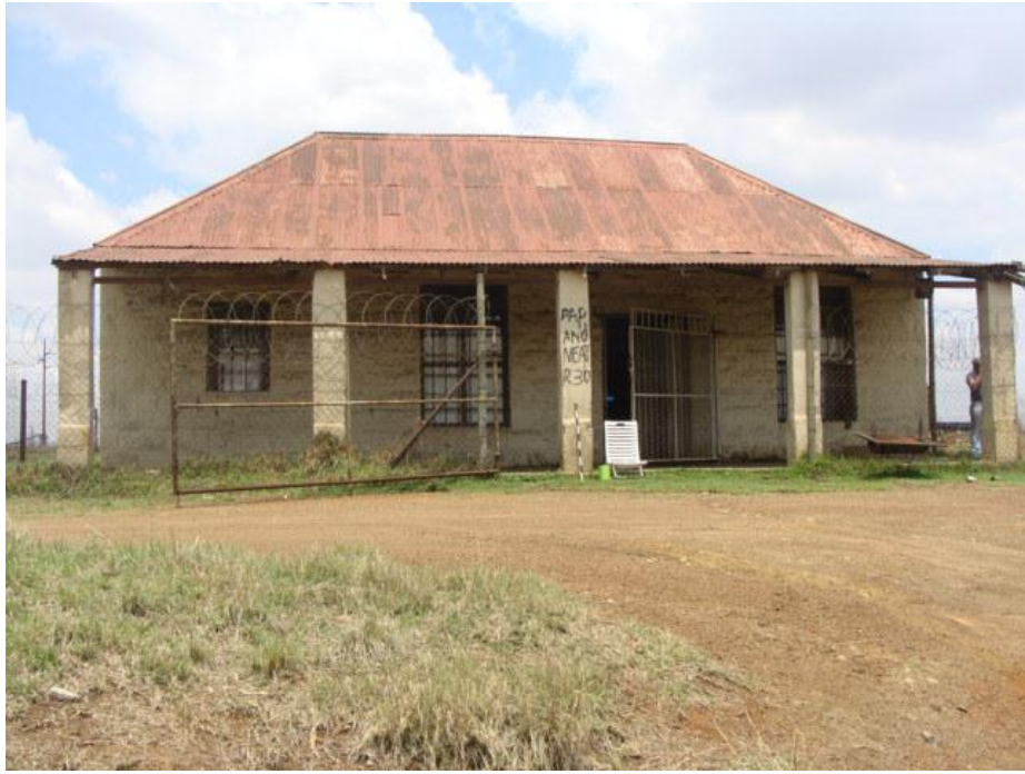
Figure 25 Front (northern) façade.
