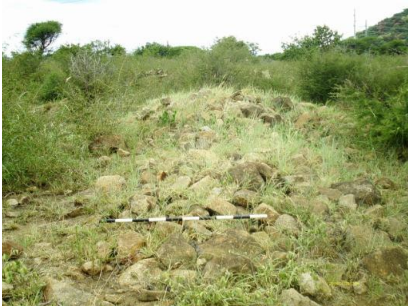
Figure 83: Collapsed stone wall and heaps of stone.
