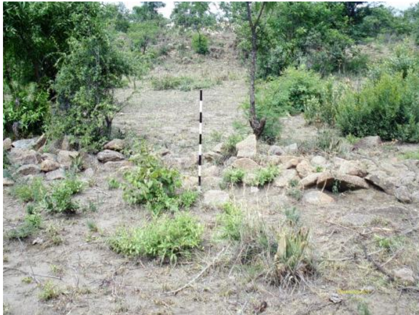
Figure 88: Another collapsed wall.
