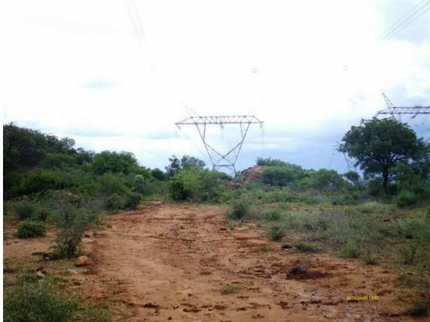
Figure 26: Road and Power line going through site.
