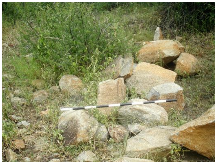
Figure74: Collapsed stone wall found on site.
