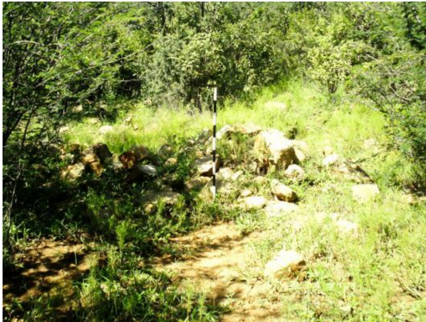
Figure 103: Broken stone wall.
