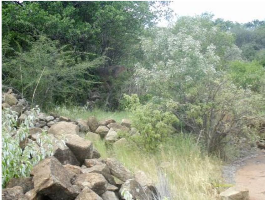
Figure 77: Stone walls covered by vegetation.
