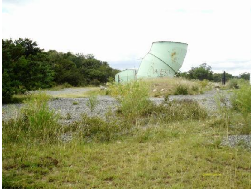
Figure 94: Mine vent in front of site.
