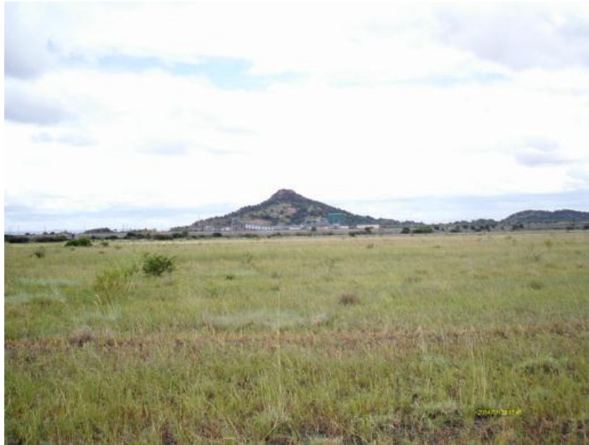
Figure 2: General view of site 1 with the Siphumelele 2 Mine shaft in the background.
