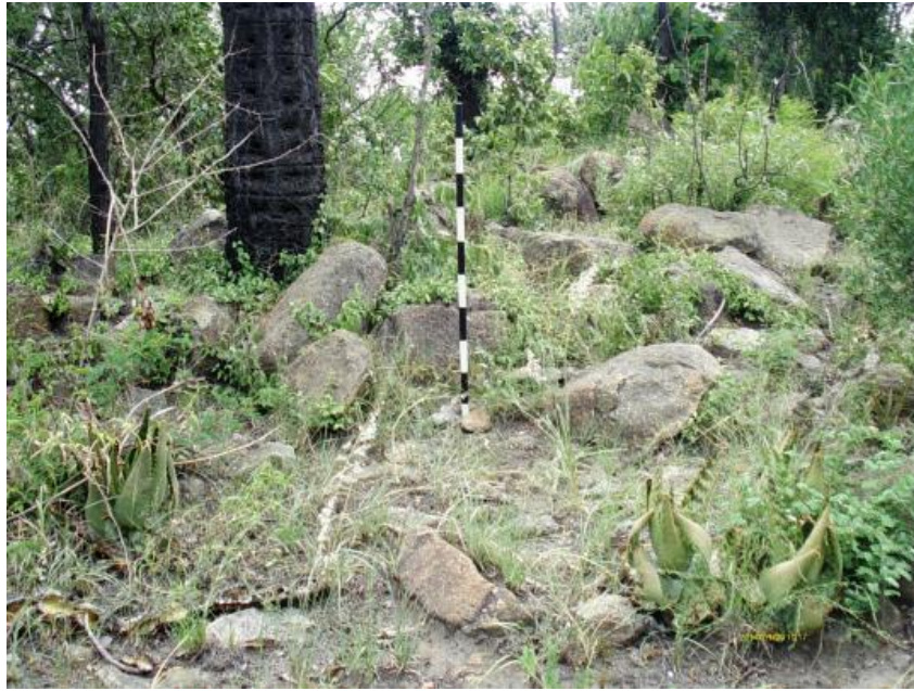
Figure 92: Collapsed stone wall.
