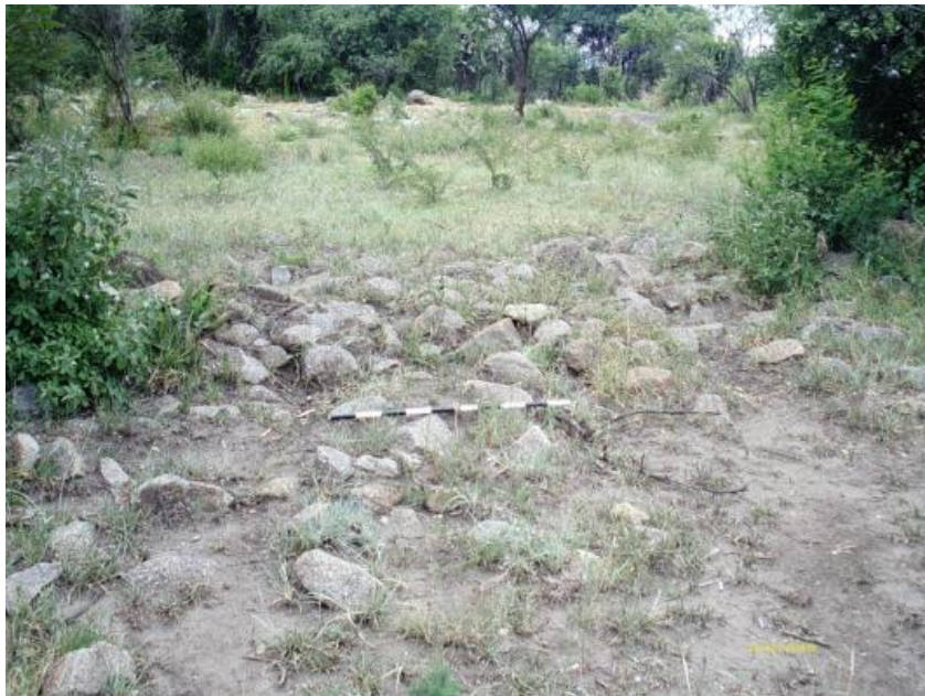
Figure 97: Collapsed stone wall.
