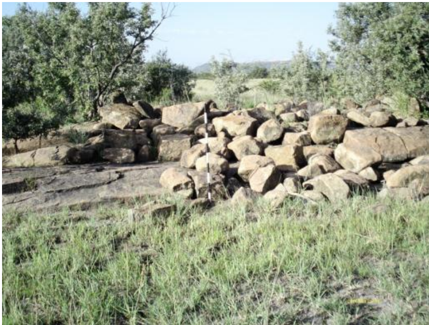
Figure 38: Collapsed on a heap of stones
