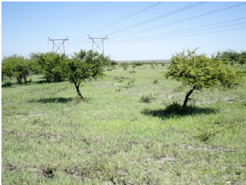
Figure 93: Power line found on the northern part of the site.
