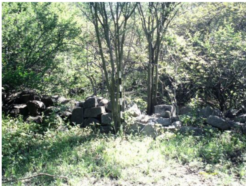
Figure 128: Overgrown stone wall.
