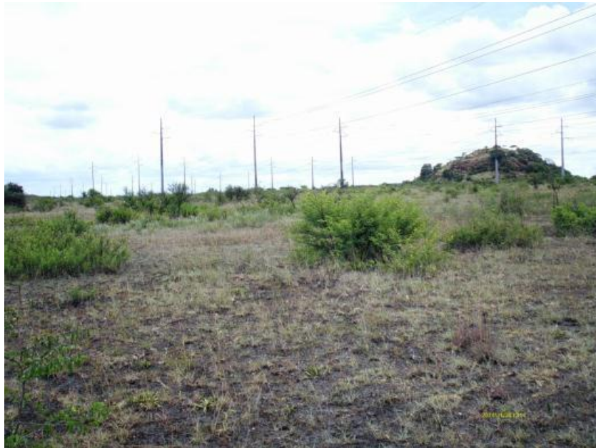
Figure 60: General view of the site with power lines running along the site.
