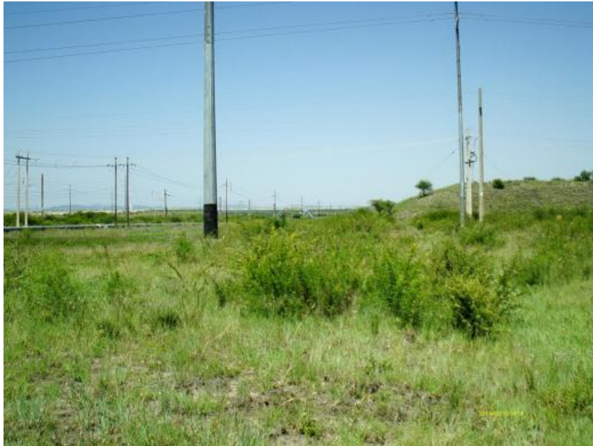
Figure 64: The site is next to a mine heap, pipe line and a power line.
