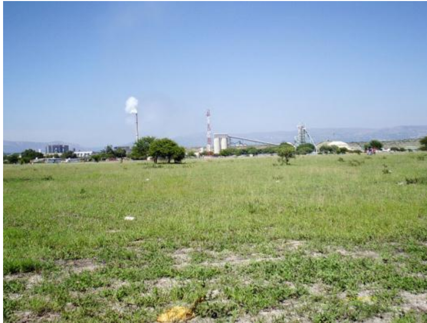
Figure 90: General view of the site, with the Khomonani 1 mine facility in the background.
