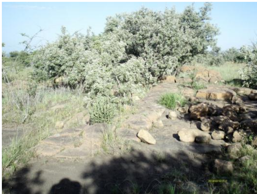
Figure 51: Heap of stones of a collapsed stone wall.
