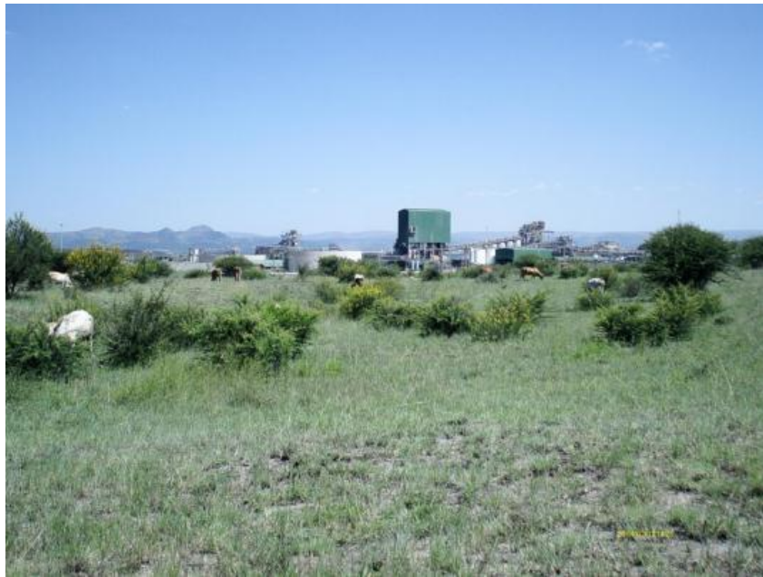
Figure 70: View of the site with the Western Limb Retreatment Plant and Concentrator in the background.
