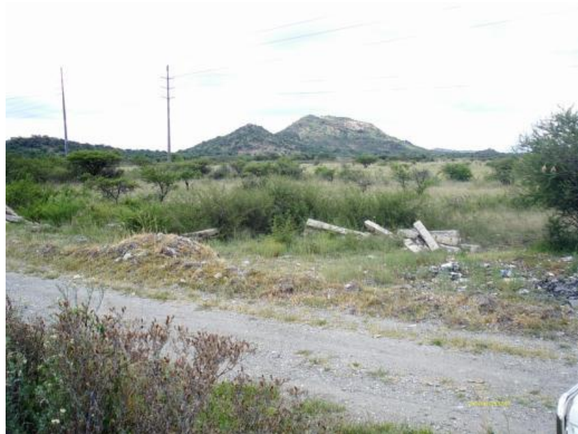
Figure 11: Unpaved road next to site. Concrete slabs indicating disturbance of the area can be seen lying next to the road.
