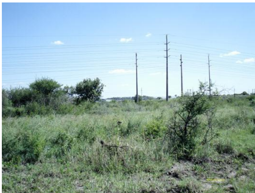
Figure 42: Power lines next to the site.
