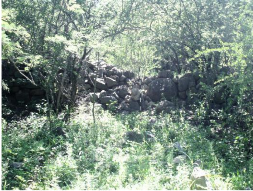
Figure 149: Overgrown semi-circular stone wall.
