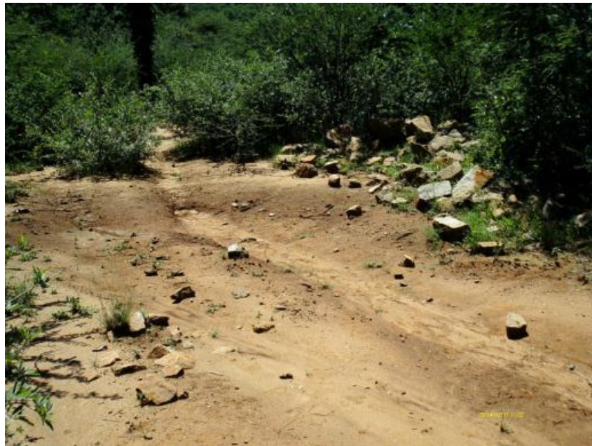
Figure 108: Broken stone wall and an unpaved road going through the feature.
