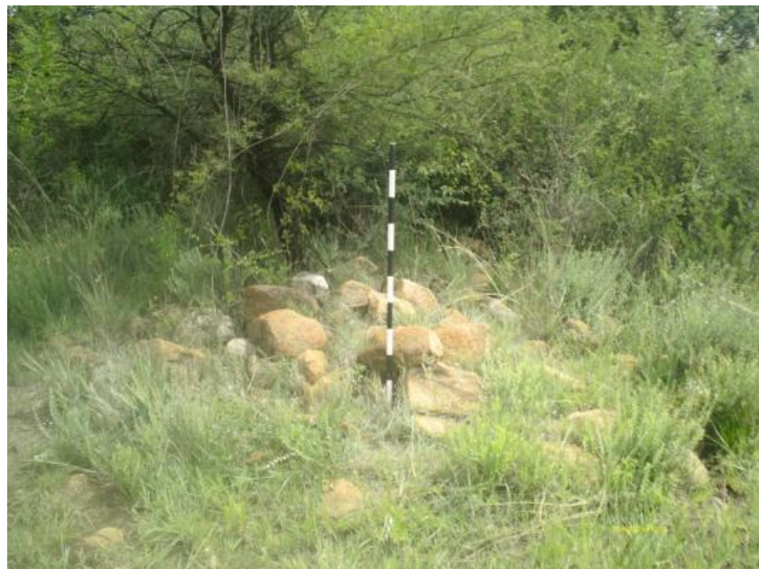
Figure 15: Collapsed stone wall.
