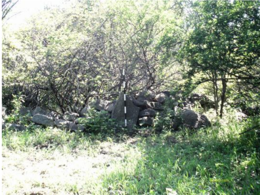
Figure 129: Another overgrown stone wall.
