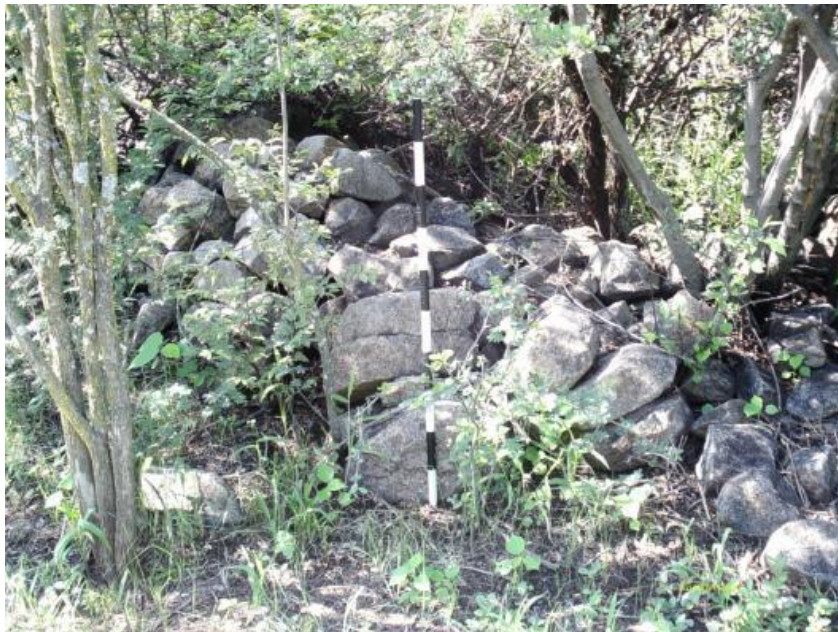
Figure 150: Walling found on site.
