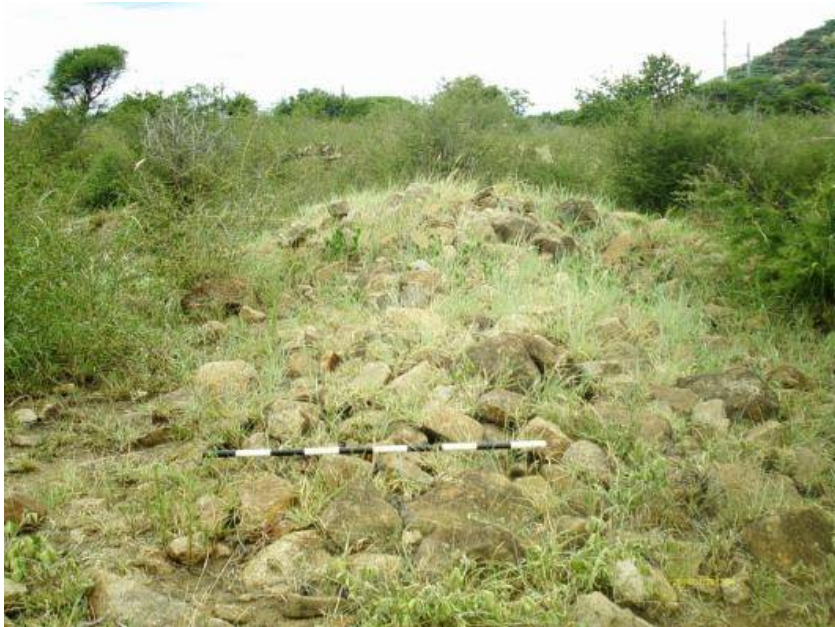
Figure 83: Collapsed stone wall and heaps of stone.
