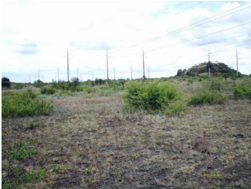
Figure 60: General view of the site with power lines running along the site.
