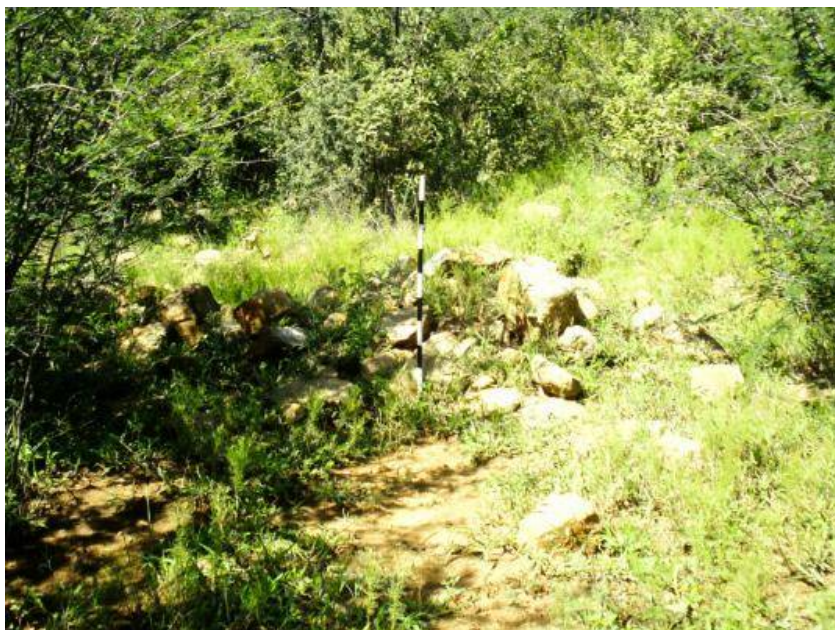
Figure 103: Broken stone wall.
