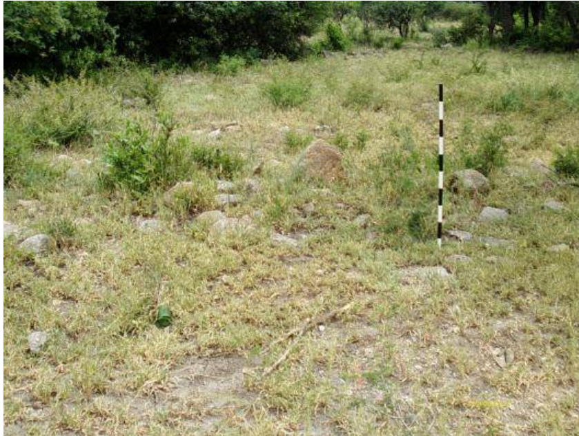
Figure 98: Another collapsed stone wall on site.
