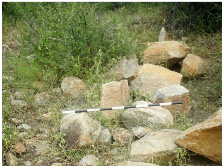
Figure74: Collapsed stone wall found on site.
