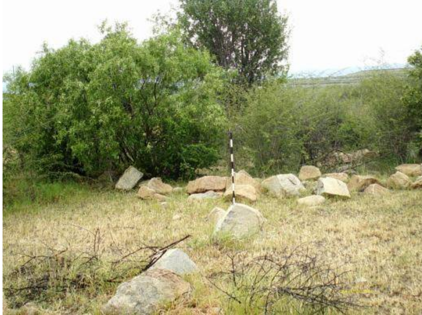
Figure 54: Collapsed stone wall.
