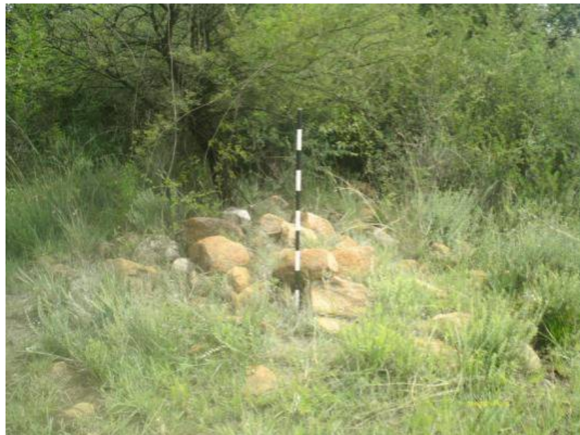
Figure 15: Collapsed stone wall.
