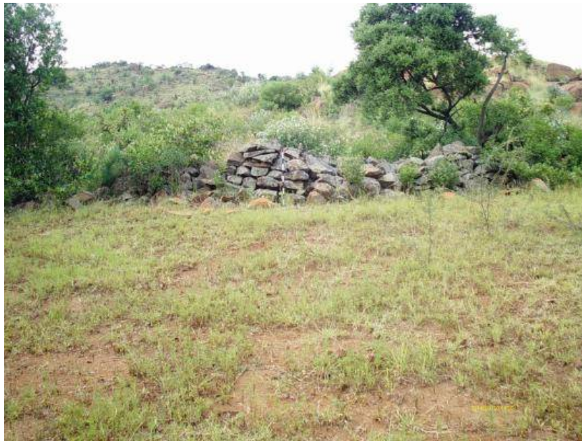
Figure 95: Stone wall covered by vegetation.
