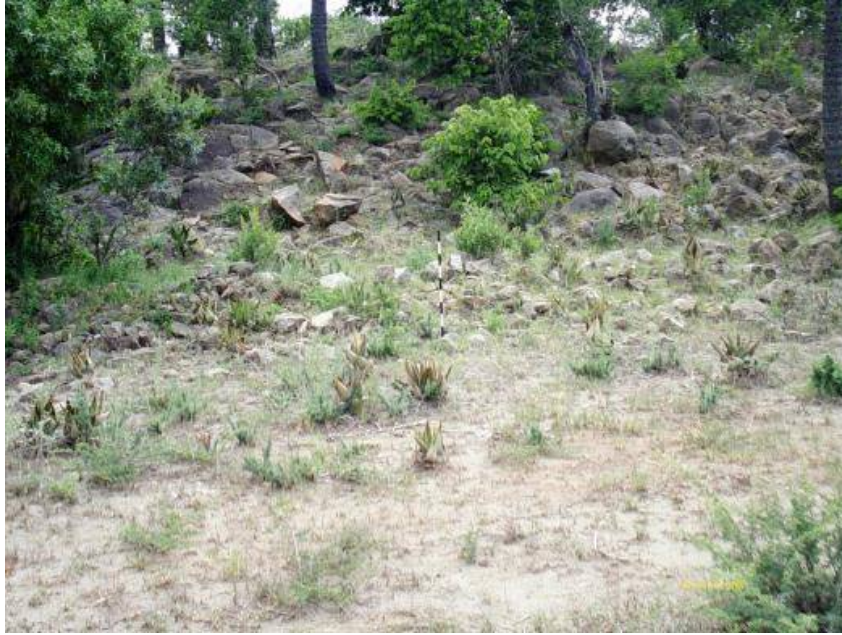
Figure 87: Collapsed wall near a small hill.
