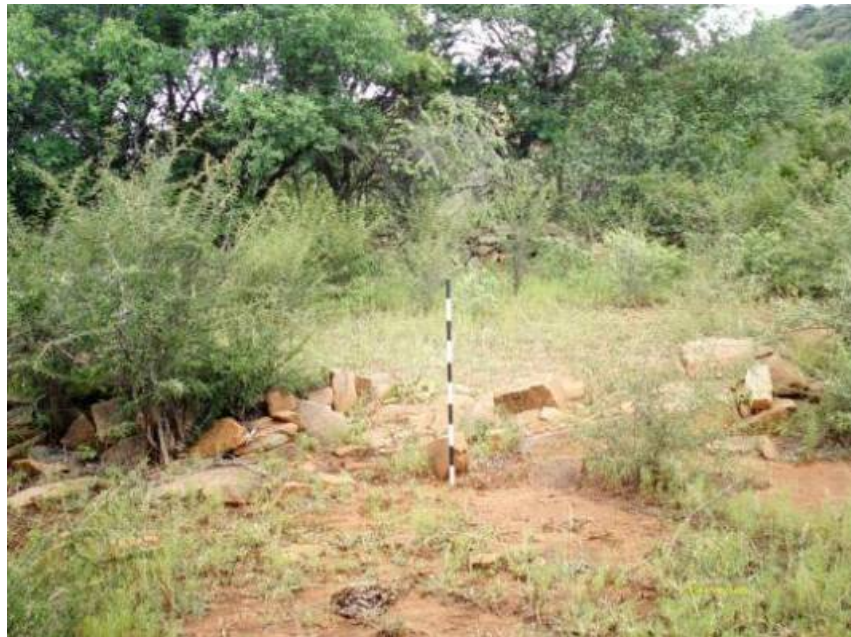
Figure 25: Collapsed stone wall.
