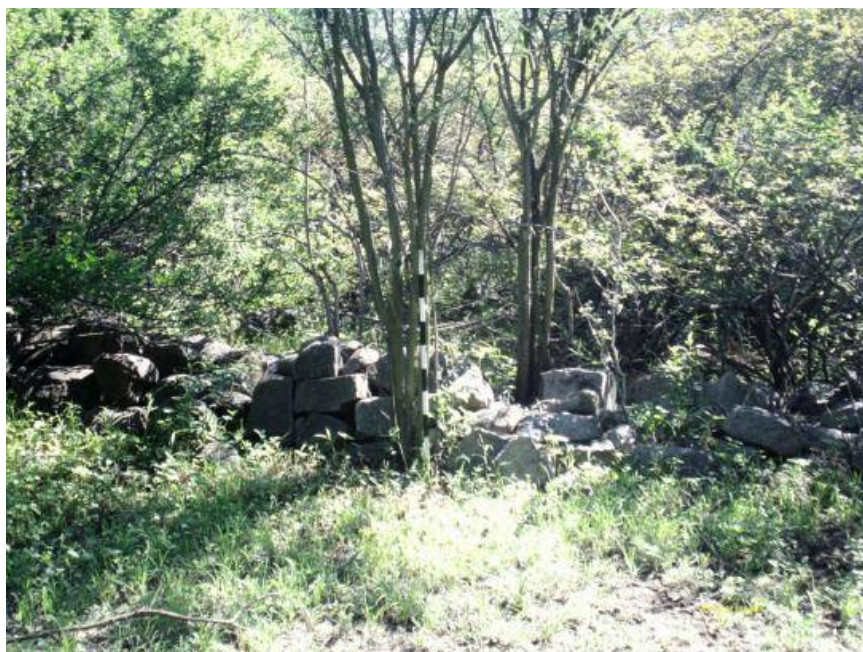
Figure 128: Overgrown stone wall.
