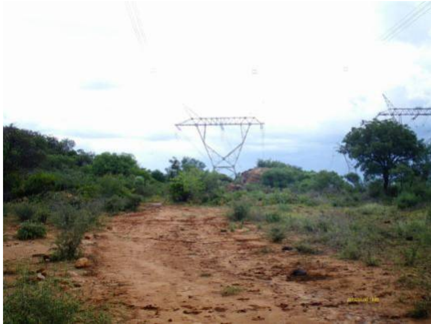
Figure 26: Road and Power line going through site.
