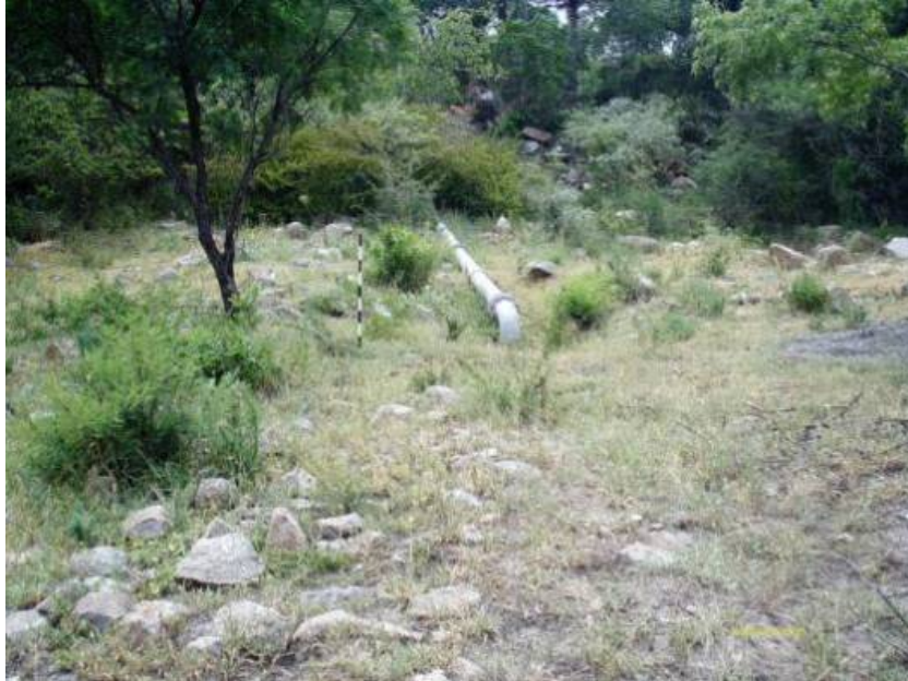
Figure 96: View of the site with pipe line in the middle of the site.
