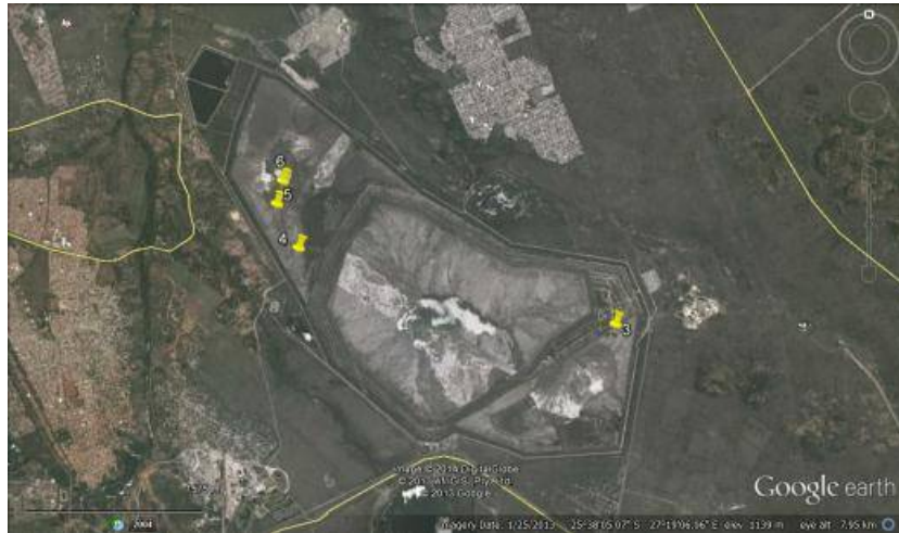
Figure 6: Google Earth image showing the sites located in the Paardekraal Tailings Storage Facility
