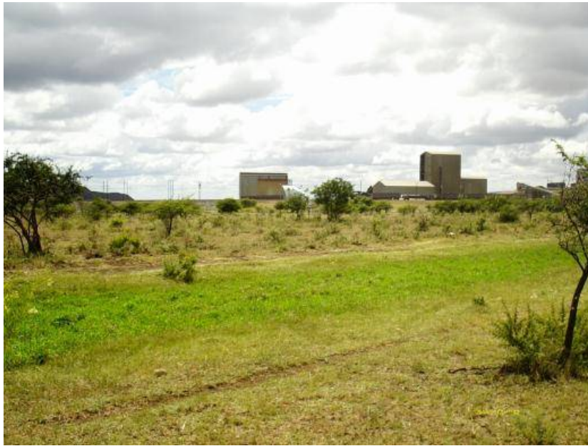
Figure 85: Siphumelele Mine close to the site.
