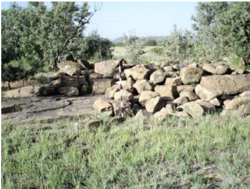
Figure 38: Collapsed on a heap of stones
