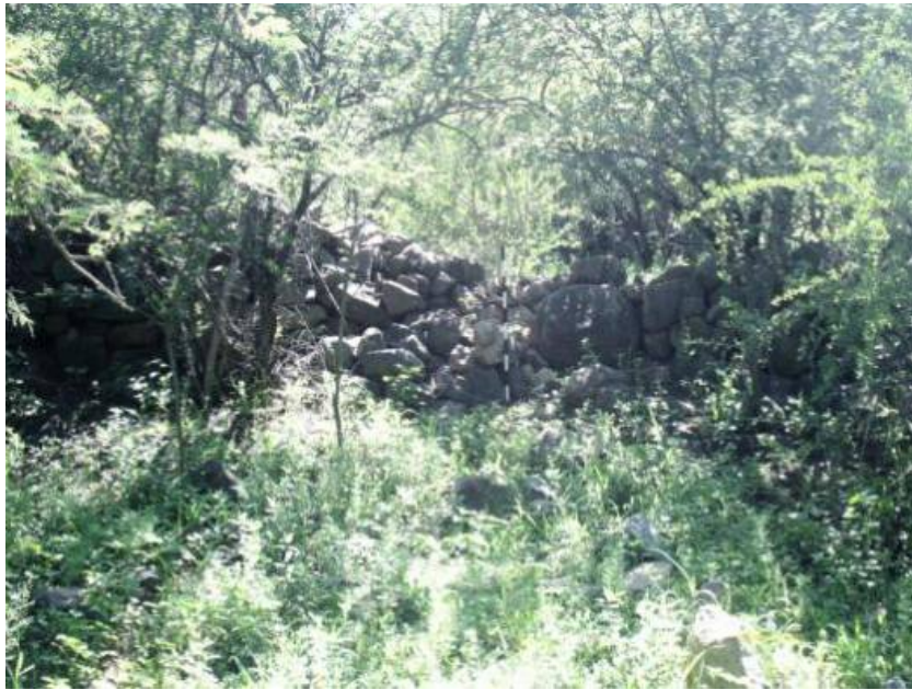
Figure 149: Overgrown semi-circular stone wall.
