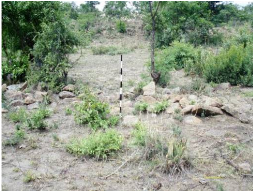
Figure 88: Another collapsed wall.
