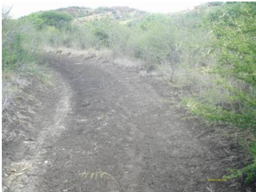
Figure 35: Unpaved road going through the site.
