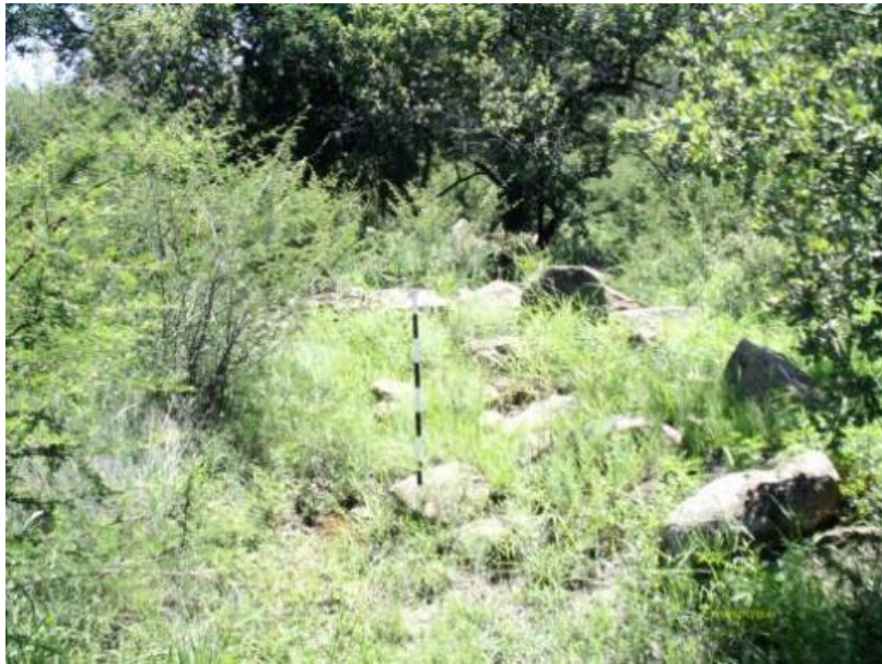
Figure 1: A collapsed and low stone wall.
