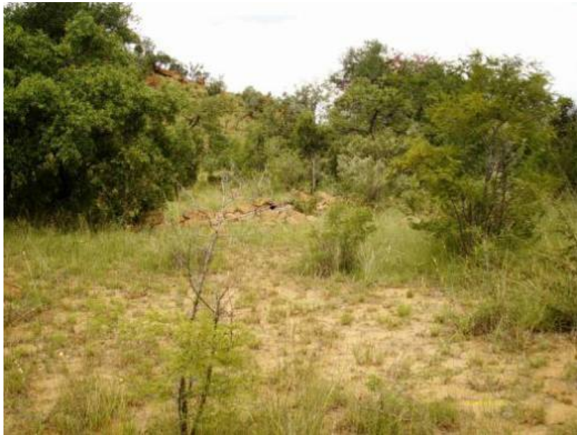
Figure 106: Collapsed stone wall.
