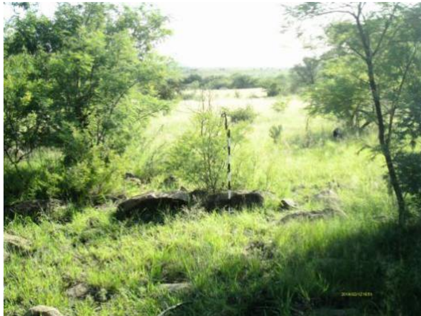
Figure 12: Low and collapsed stone wall on site.
