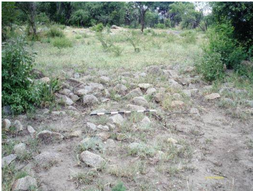
Figure 97: Collapsed stone wall.
