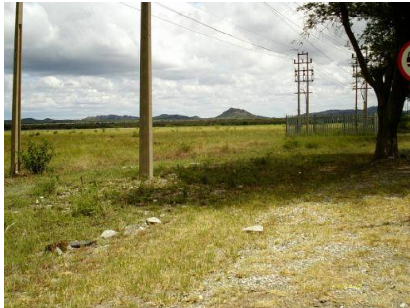
Figure 3: Power lines running along the site.
