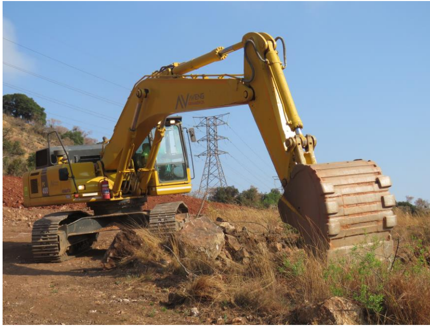
Figure 33: The excavator that was used in the demolition of the site.
