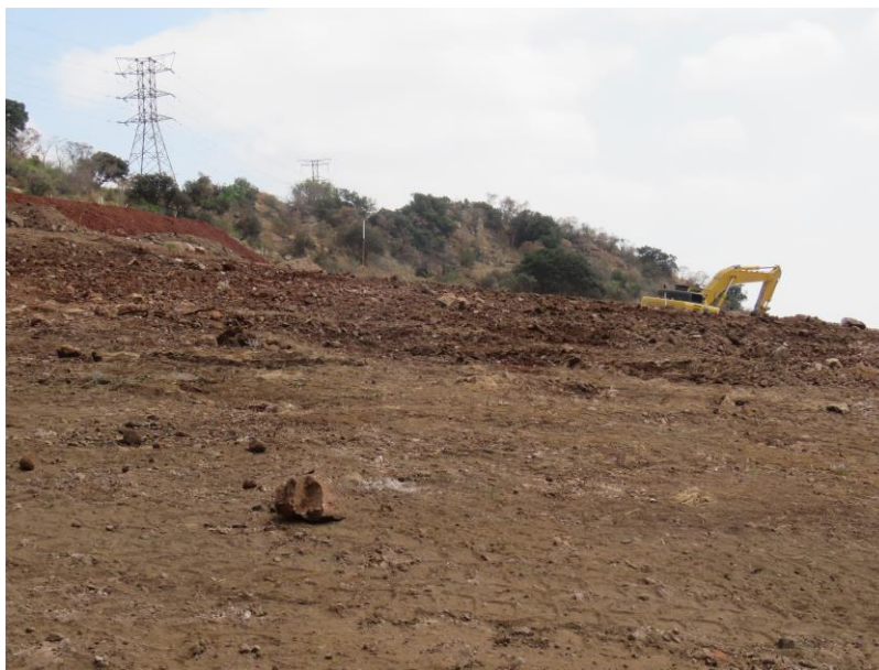
Figure 34: The site after the demolition of the blockhouse.
