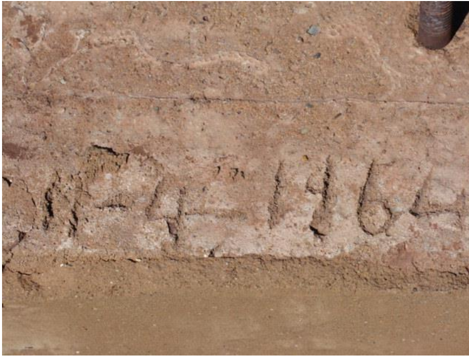
FIGURE 36: (11-4-1964) INDICATED ON THE BUILDING.
