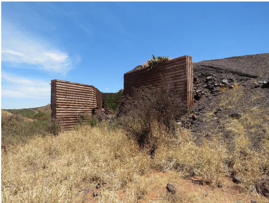
FIGURE 39: REMAINS OF AN ORE LOADING BAY, SITE NO. 14.
