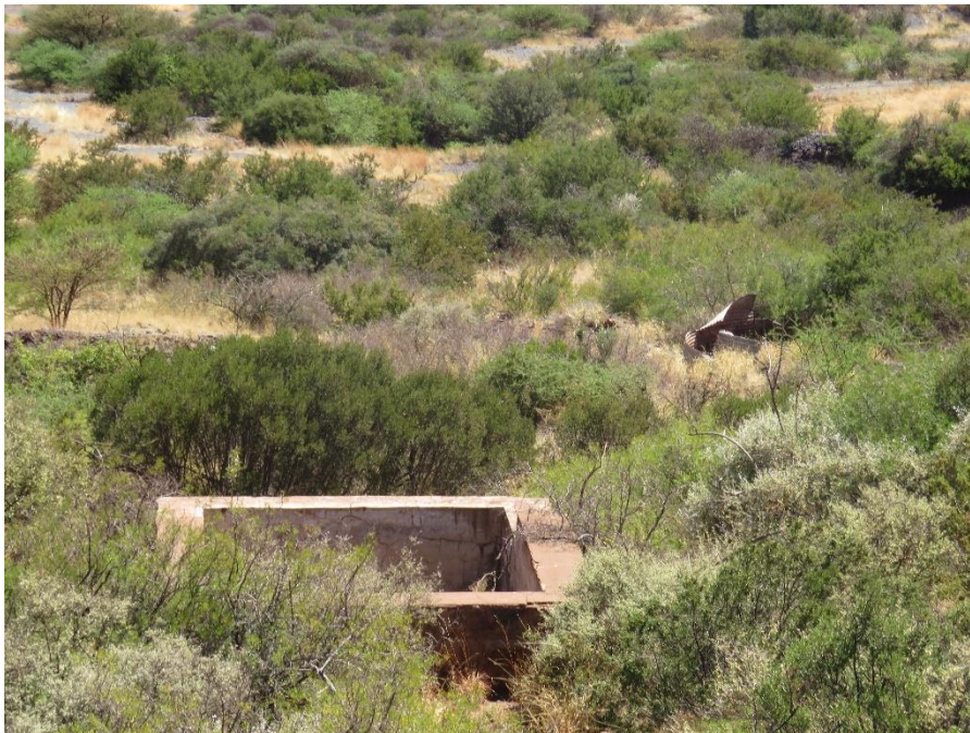
FIGURE 57: BUILDING ASSOCIATED WITH LOADING PLATFORM.
