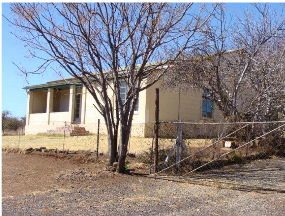
FIGURE 32: HOUSE NUMBER 1 AT SITE NUMBER 4.
