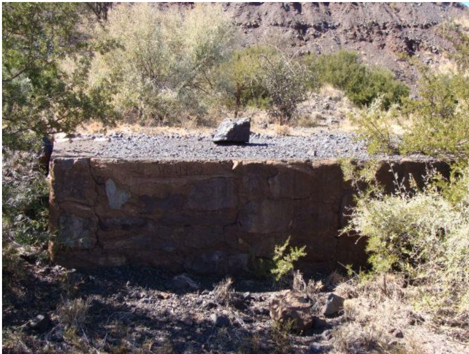
FIGURE 42: THE LOADING PLATFORM.
