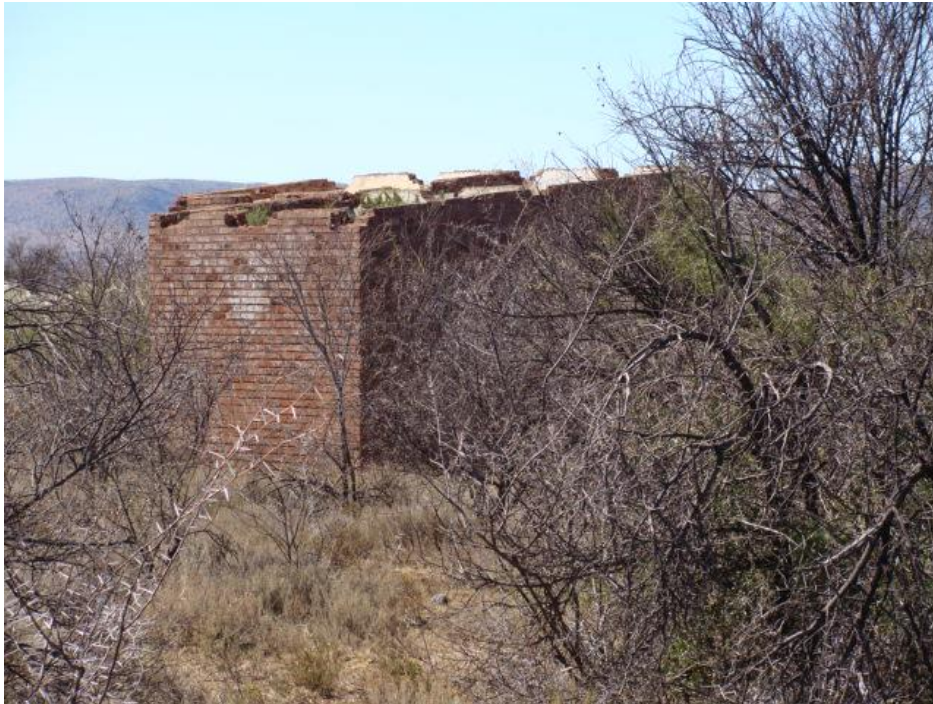
FIGURE 52: REMAINS OF ONE OF THE BUILDINGS AT SITE NUMBER 11.
