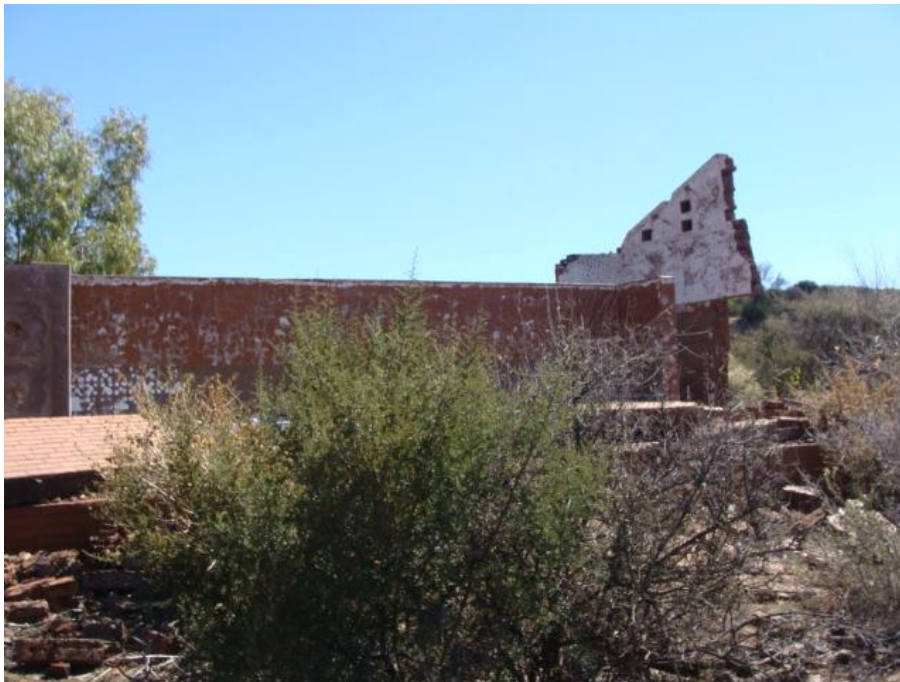
FIGURE 46: REMAINS OF THE TOILET BUILDING.
