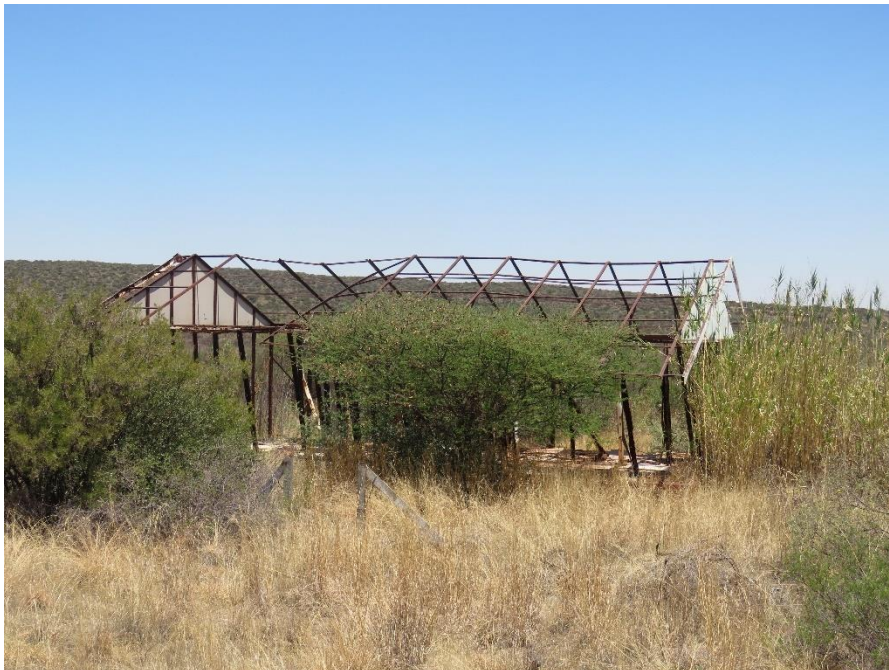
FIGURE 59: STEEL FRAME OF A RAILWAY BUILDING.
