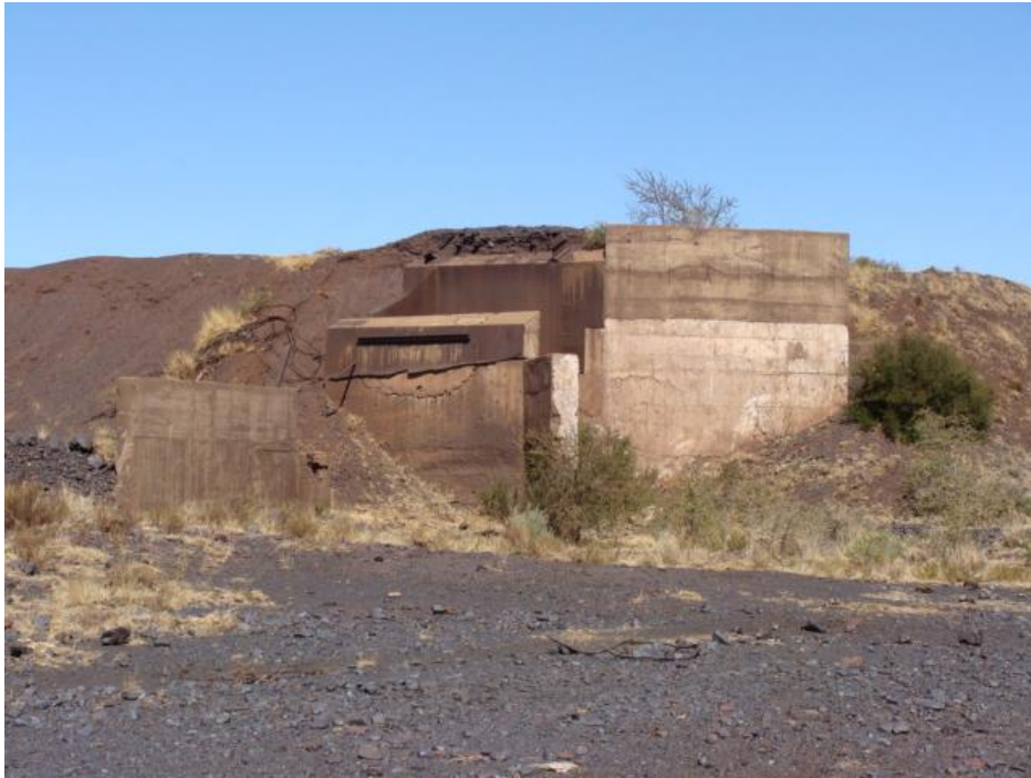
FIGURE 38: REMAINS OF AN ORE LOADING BAY, SITE NO. 7.
