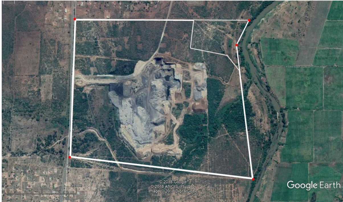
Figure 5: Detailed view of the applicable area. Note the large-scale disturbance by mining activities.
