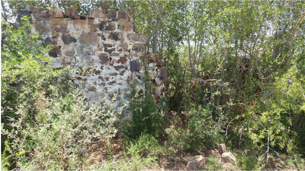
Figure 20: Another view of the same building.
