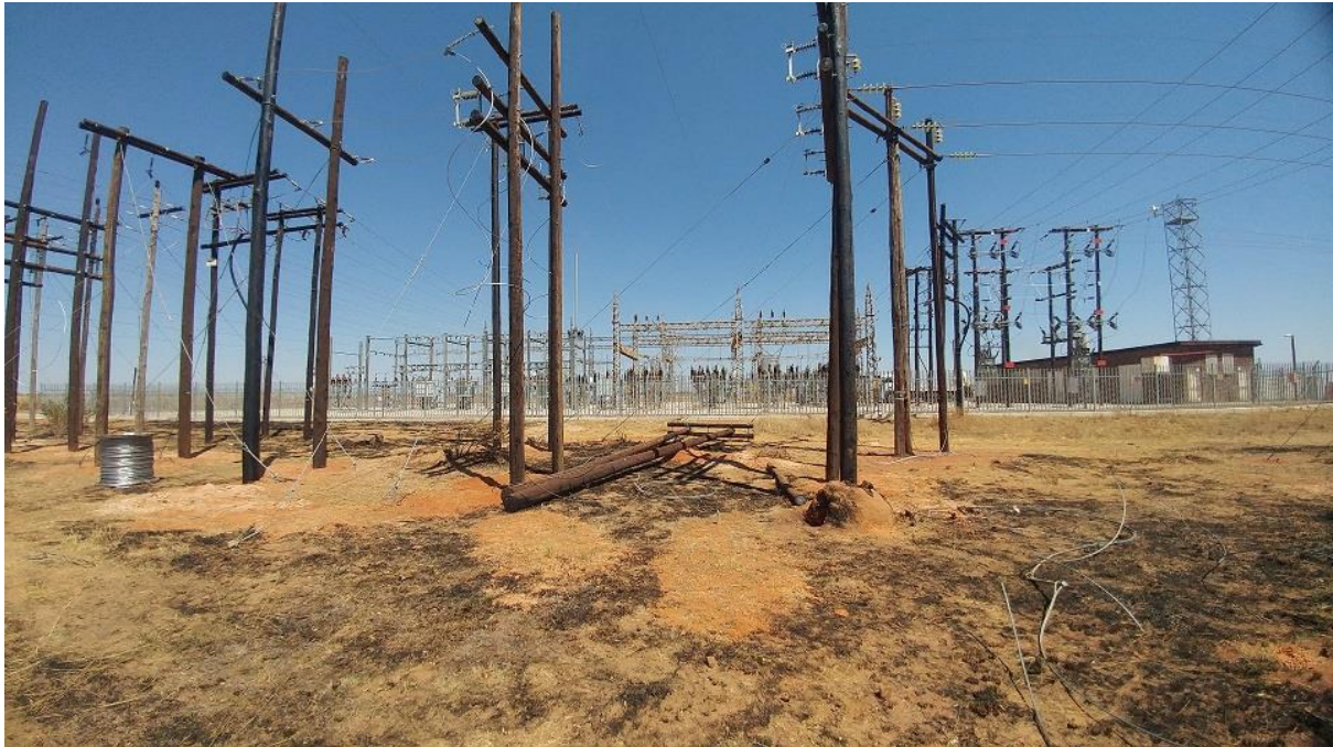
FIGURE 5: POWER LINE IN THE SURVEYED AREA.
