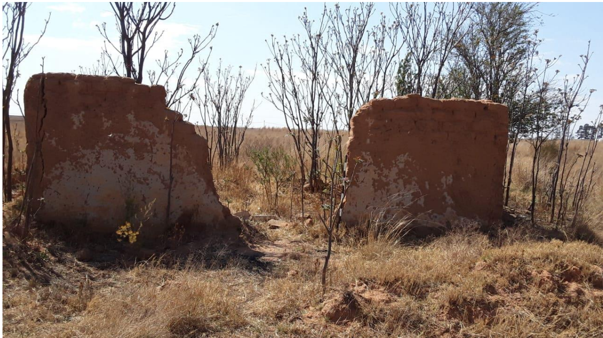
FIGURE 66: GENERAL VIEW AT THE STRUCTURE AT SITE NO. 20.
