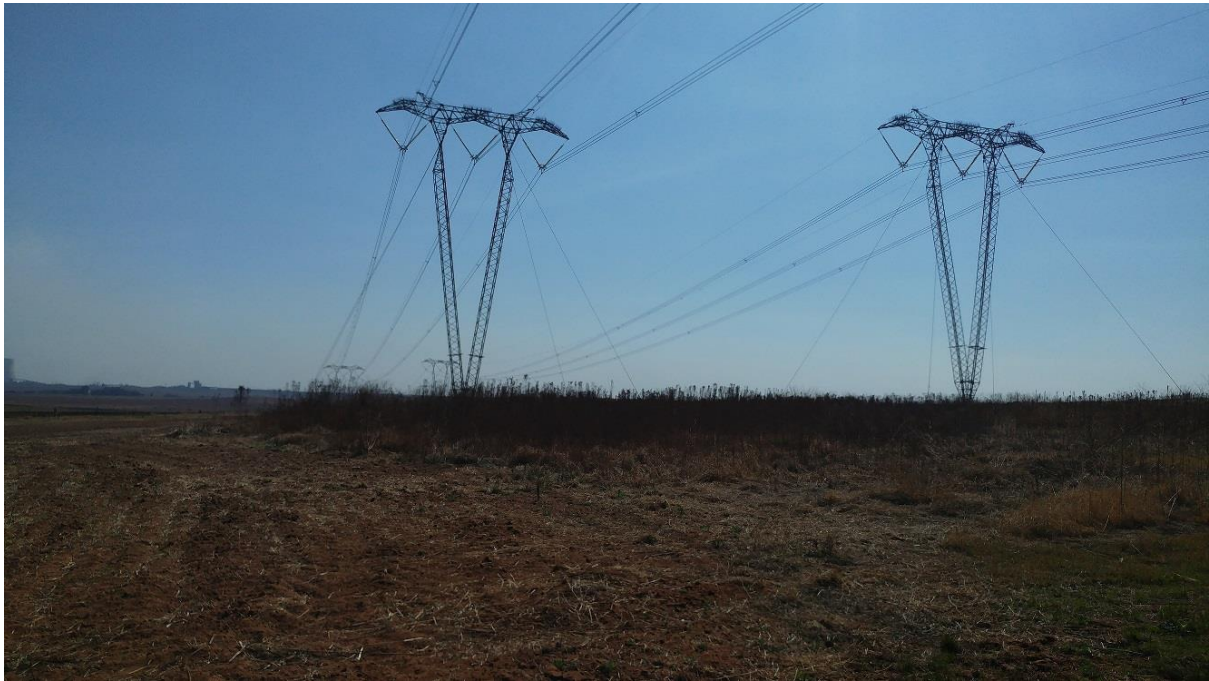
FIGURE 16: PIONEER VEGETATION GROWING UNDER POWER LINES IN THE SURVEYED AREA.
