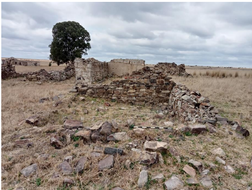
Figure 21: North facing view of stone structure 3 at site 4.
