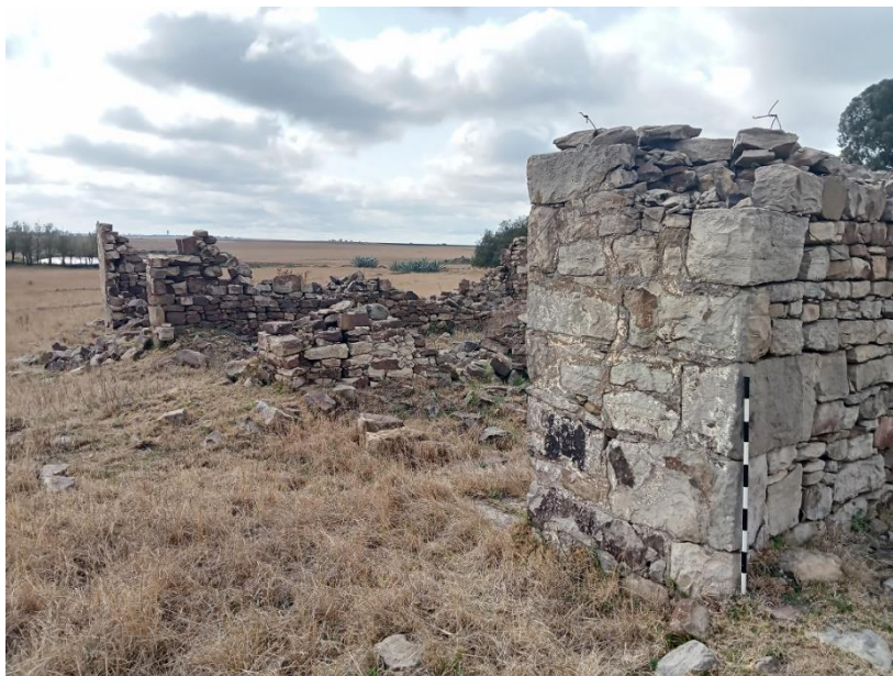
Figure 17: North facing view of structure 2 at site 4.
