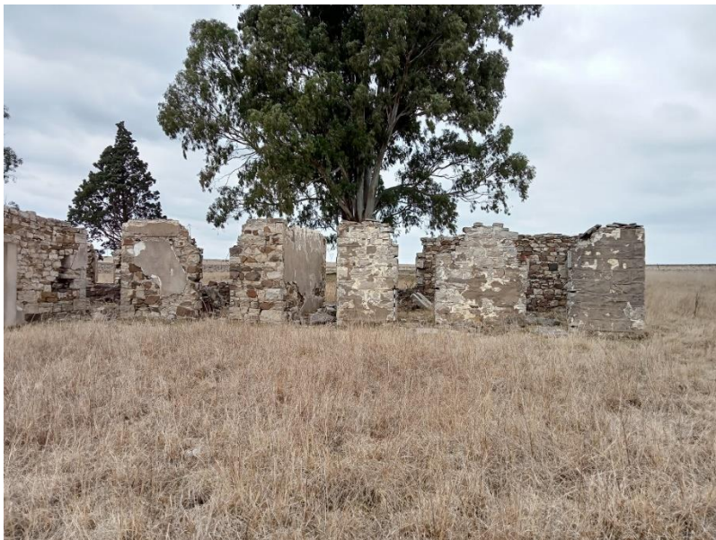
Figure 27: North facing view of utility rooms at site 5.
