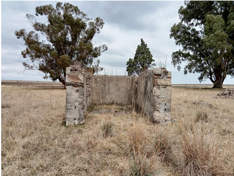
Figure 22: Northern view of structure 1 at site 5.
