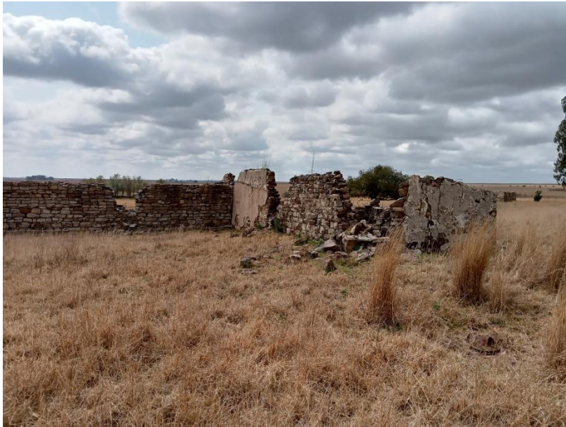
Figure 20: West facing view of structure 2 at site 4.
