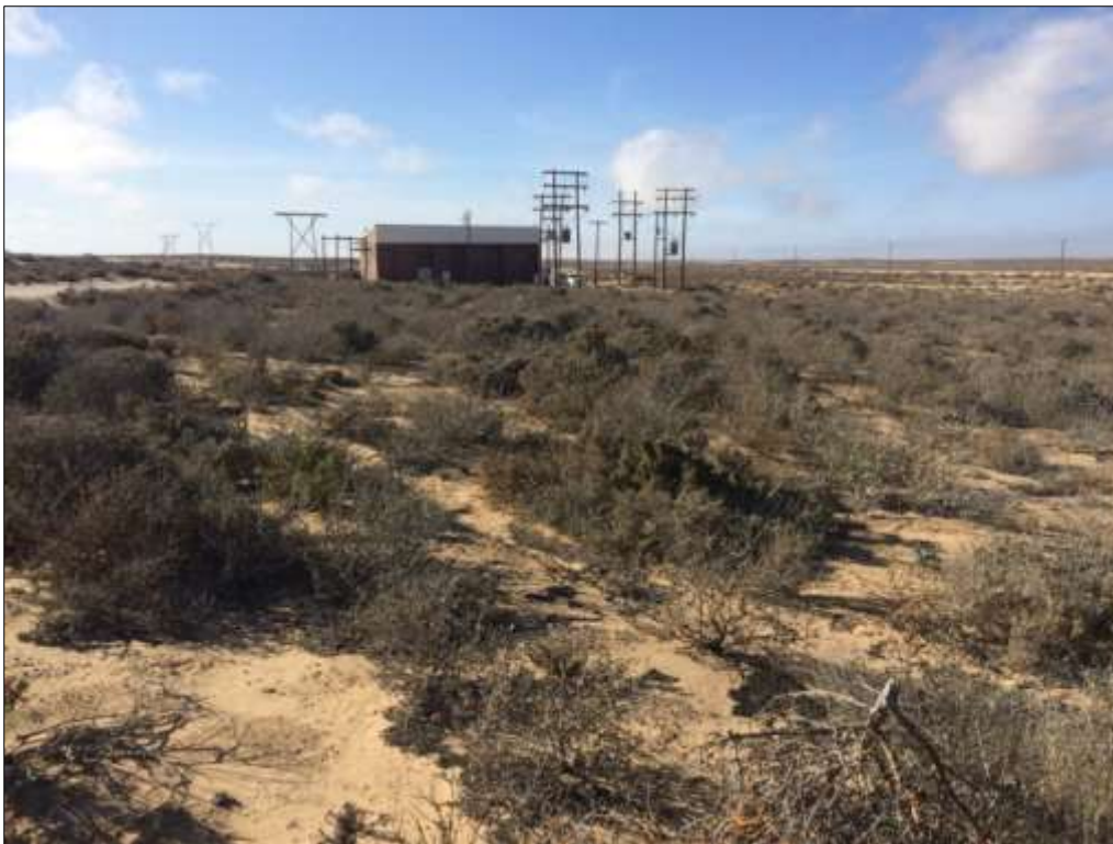
Figure 4. View of the proposed development site facing south. The Eskom Muisvlakte Substation is in the background of the plate
