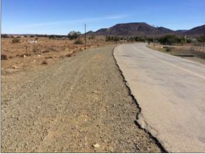
Figure 24. Proposed sewer route alongside R355 south
