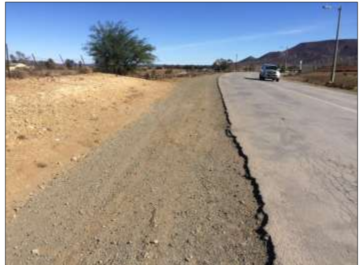
Figure 23. Proposed sewer route alongside R355 south
