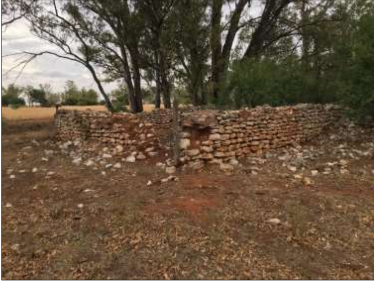
Figure 22. Historic (c. 1899) calcrete stone and mud sheep enclosure
