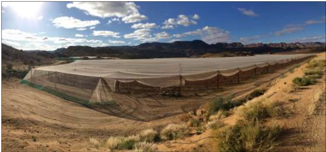
Figure 10. Area 4. View facing north west
