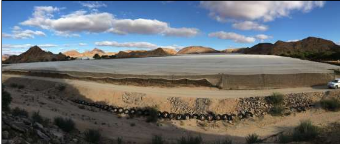
Figure 12. Area 4. View facing south east
