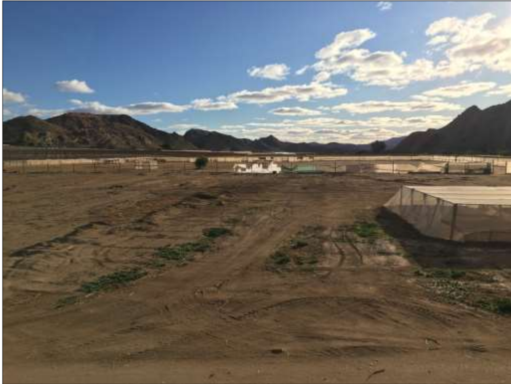
Figure 15. Area 5. View facing west
