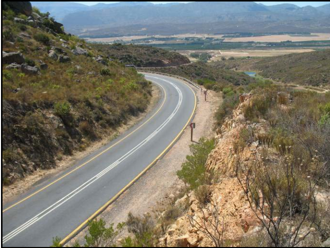
Figure 19. Sandstone outcropping to be removed
