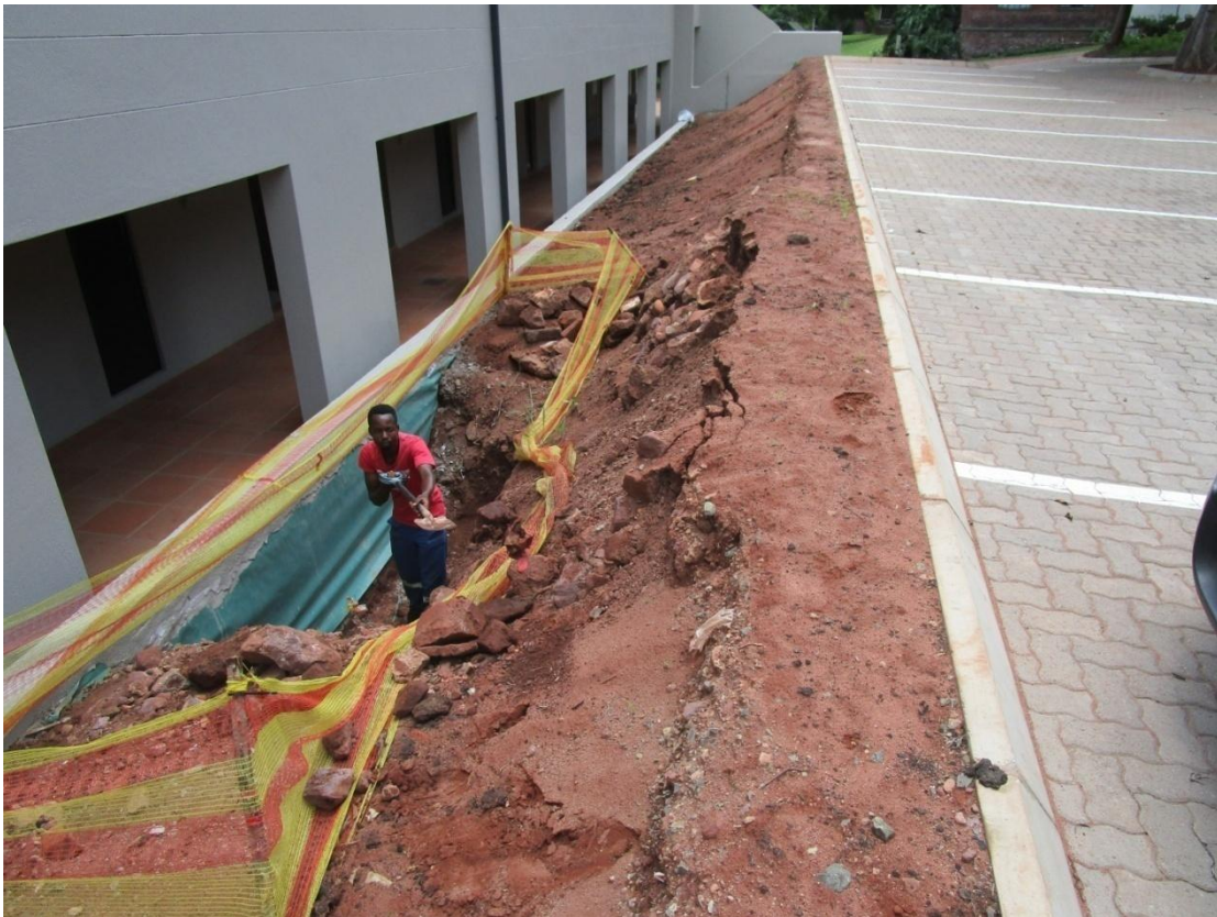
Figure 1. View of the trench being cleaned of rubble and debris.
