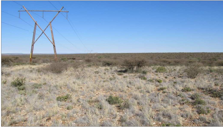
Figure 19. View facing west alongside the existing Moidraai servitude
