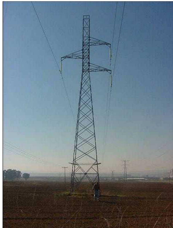
Figure 26. Example of steel lattice structure
