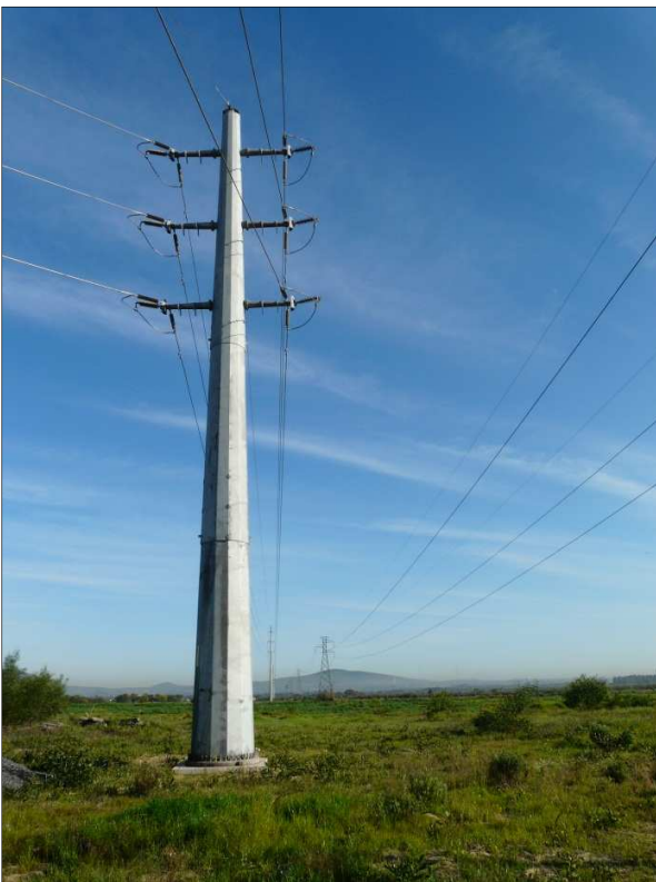
Figure 25. Example of single strain monopole
