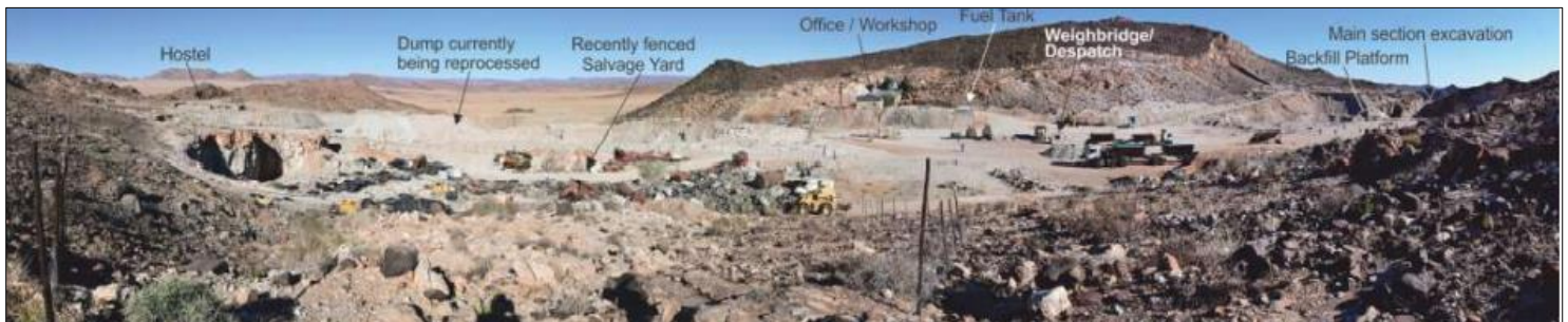
Photo 1: General view of the main excavation and logistical facility looking north, with the hostel in the west and the main excavation in the east.
