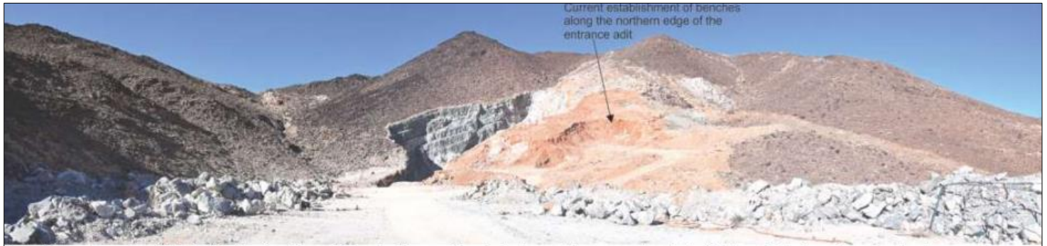
Photo 3: General overview of the Kloof Section from the north showing the recent bench development (orange area) and just off picture right is the main overburden dump seen in Photo 5.
