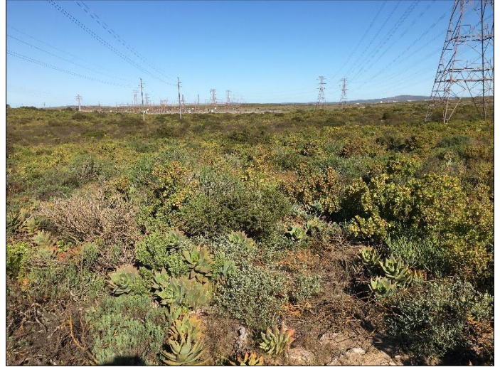
Figure 26. Route Option 3. View facing north, with the Blouwater substation in the distance.
