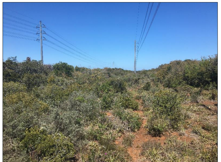
Figure 8. Zone 11, view facing south
