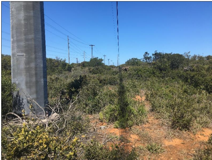
Figure 5. Zone 11, view facing south
