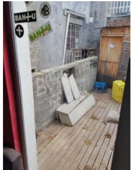
First floor deck over courtyard
