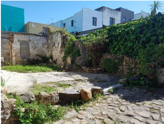
Open yard, retaining wall, public parking behind
