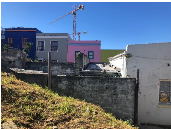
South façade backyard
