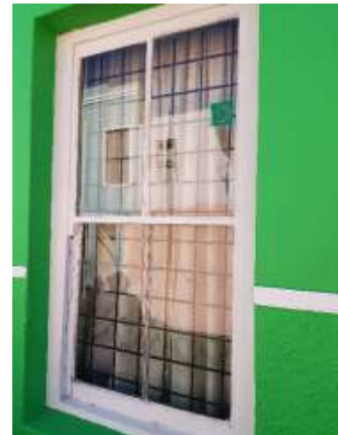
Existing sash window
