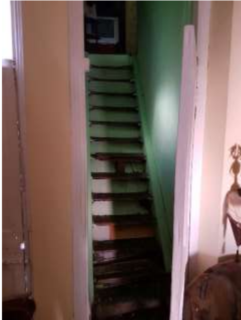
Existing stair (to be replaced)
