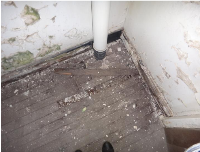
Timber infill floor to enclosed veranda.
