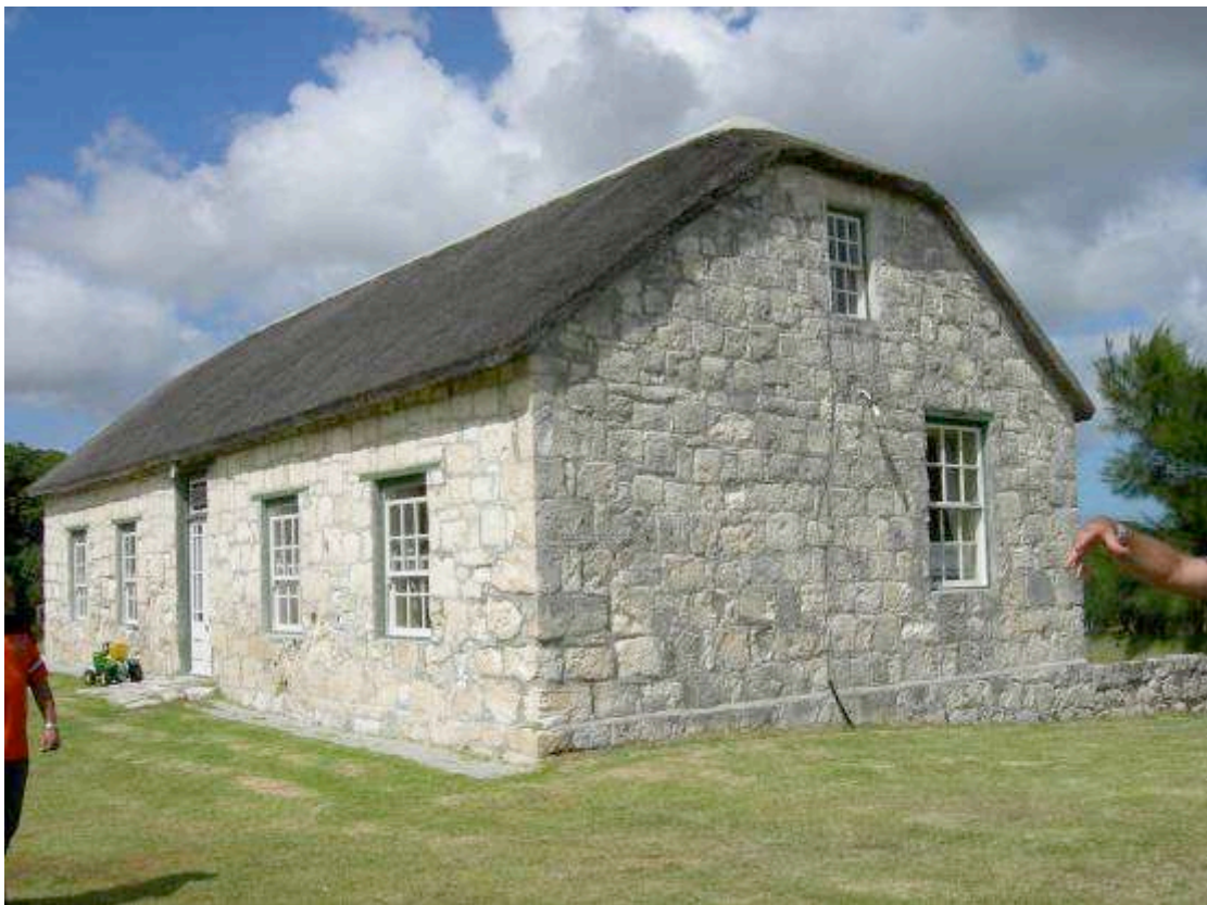
Figure 13 (below) Farm house at Groot Hagelkraal farm complex. Although recently renovated, the building contains mid-late 19 th century fabric.
