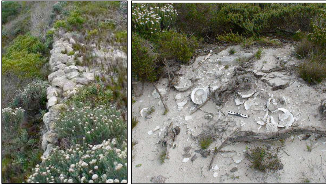
Figure 8 (above left) Historic limestone boundary wall, Bantamsklip.
