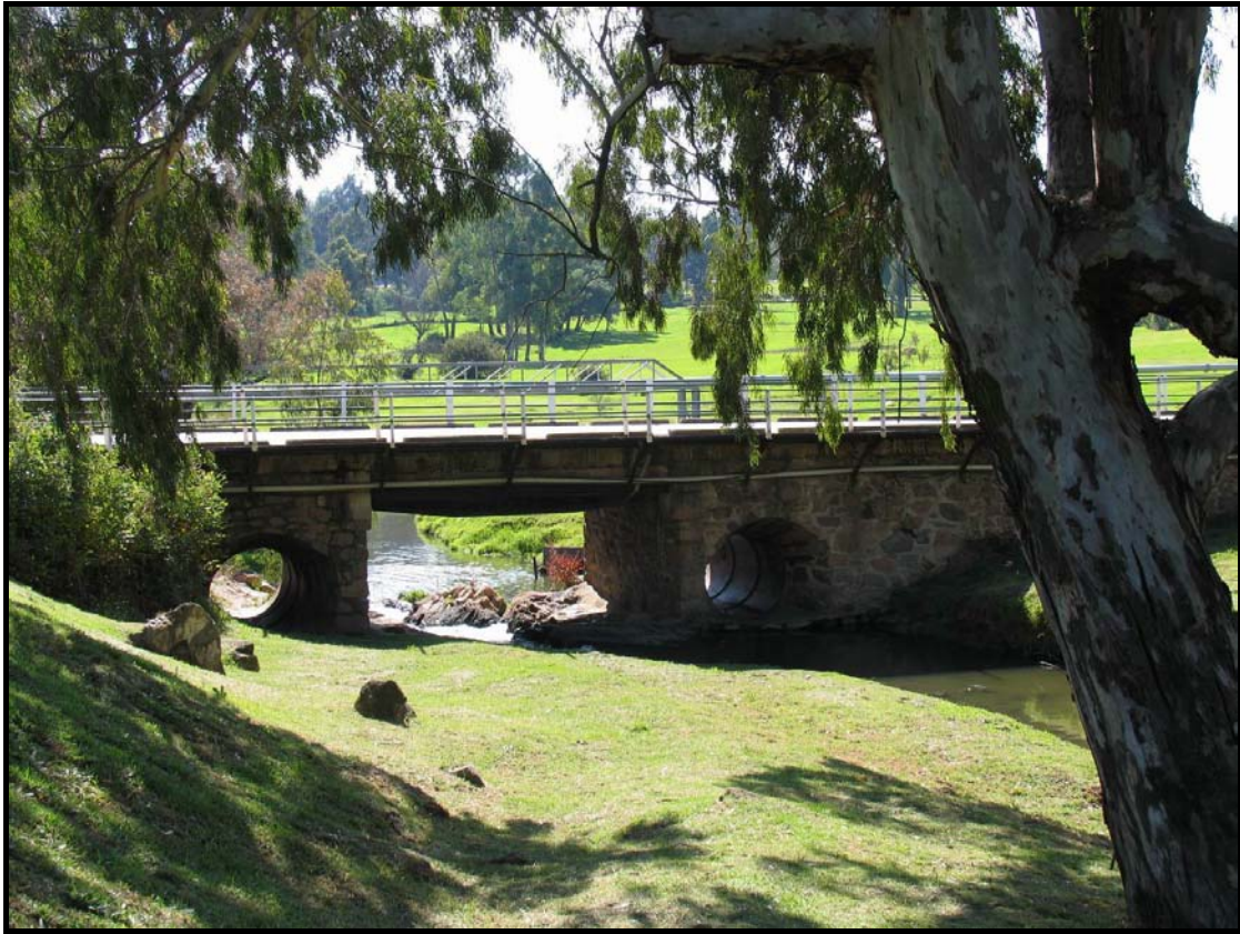
Figure 19. Old bridge built from stone (Site no 61).
