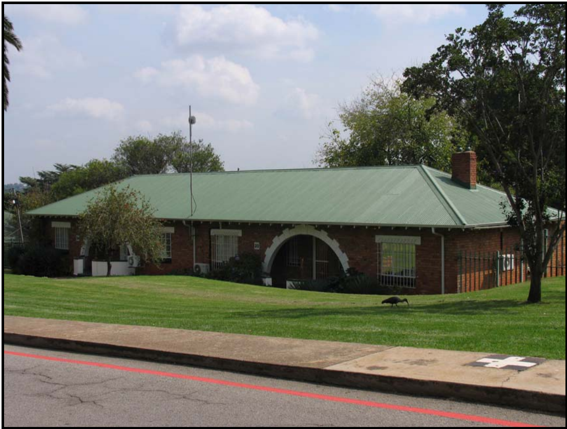
Figure 16. One of a series of semi-detached houses, dating to the 1940s and early 1950s (Site no 76).
