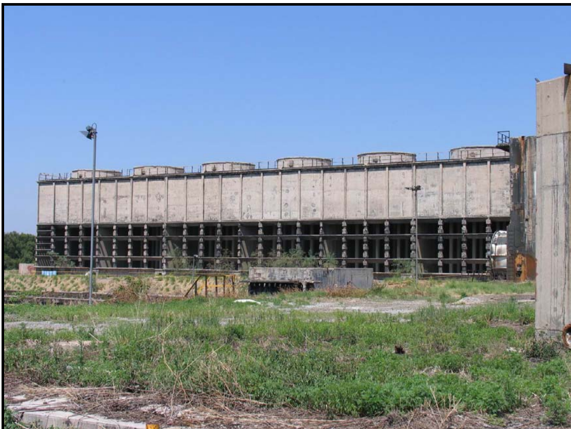
Figure 7. Old cooling plant of concrete.
