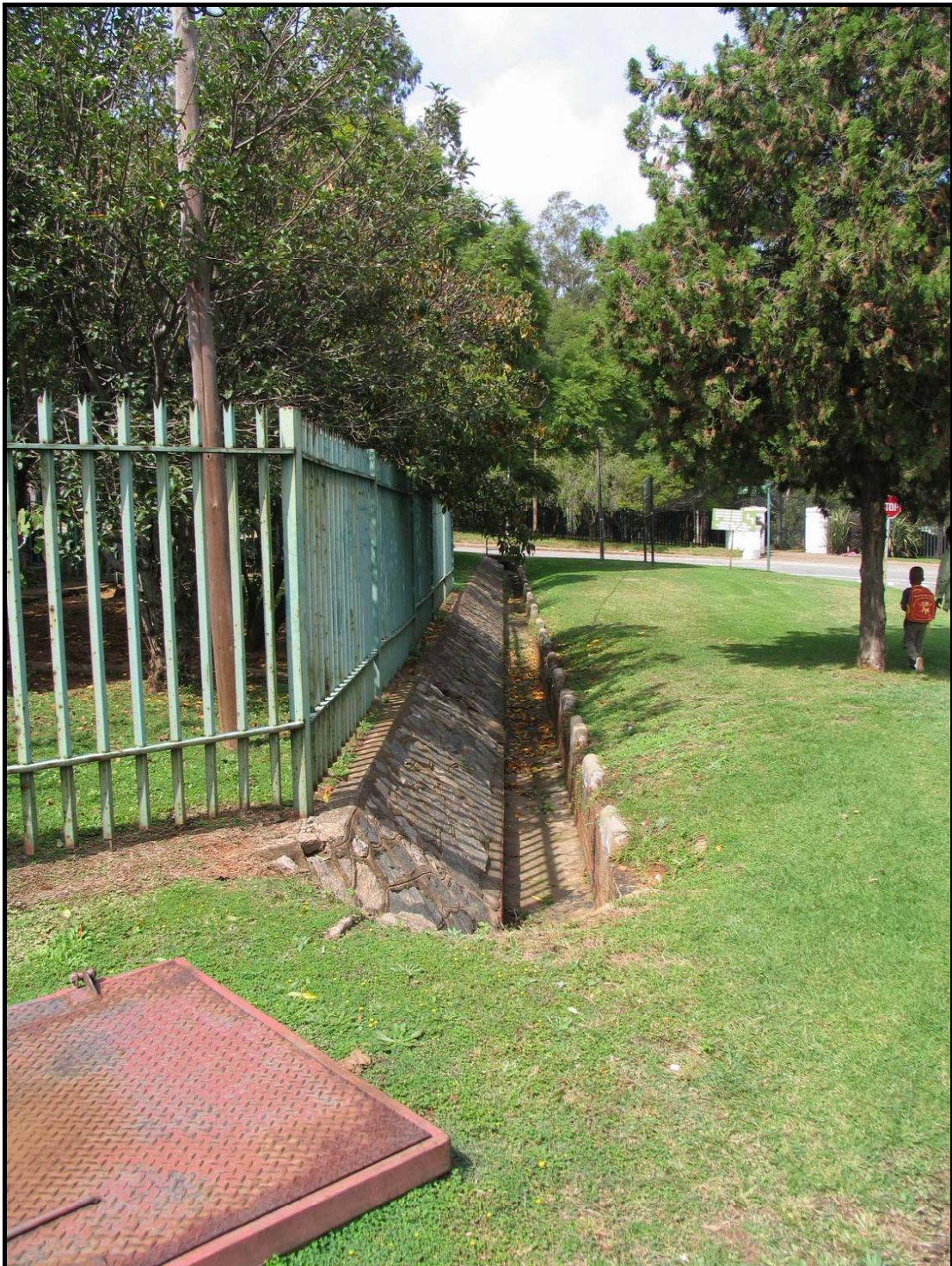
Figure 18. An old water furrow/storm water channel (Site no 79).
