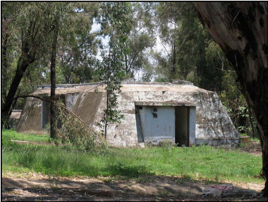
Figure 10. One of the old bunkers that dot the landscape (Site no. 75).
