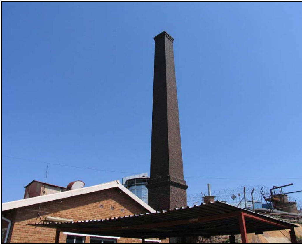
Figure 6. Old chimney built from brick, probably early 20 th century (Site no. 73).
