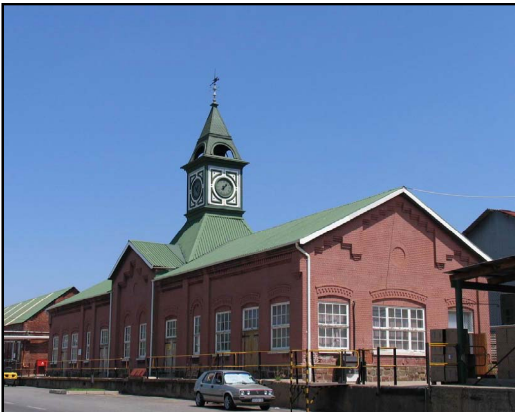
Figure 5. Clock-tower building (Site no. 74).
