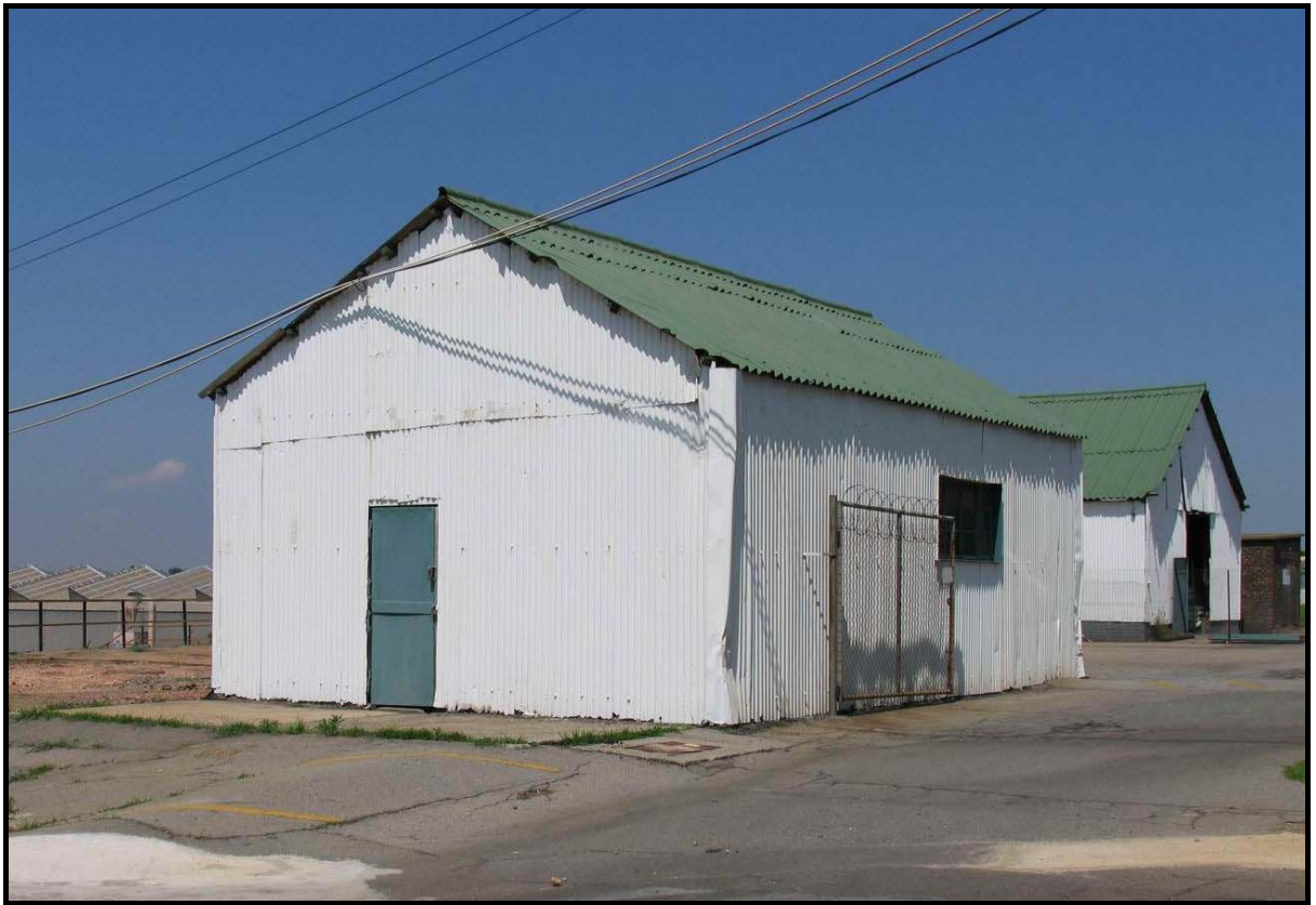
Figure 8. One of a large number of corrugated iron sheds.
