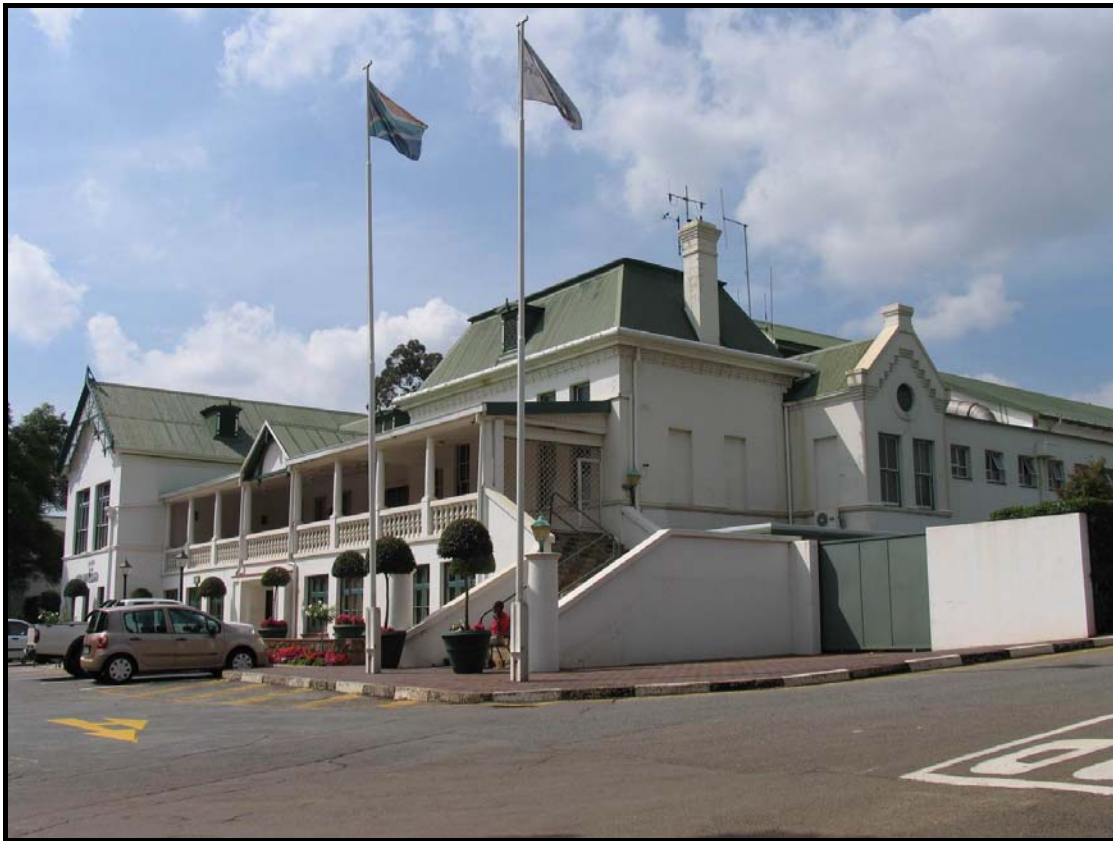
Figure 4. The main office building (Site no. 70).
