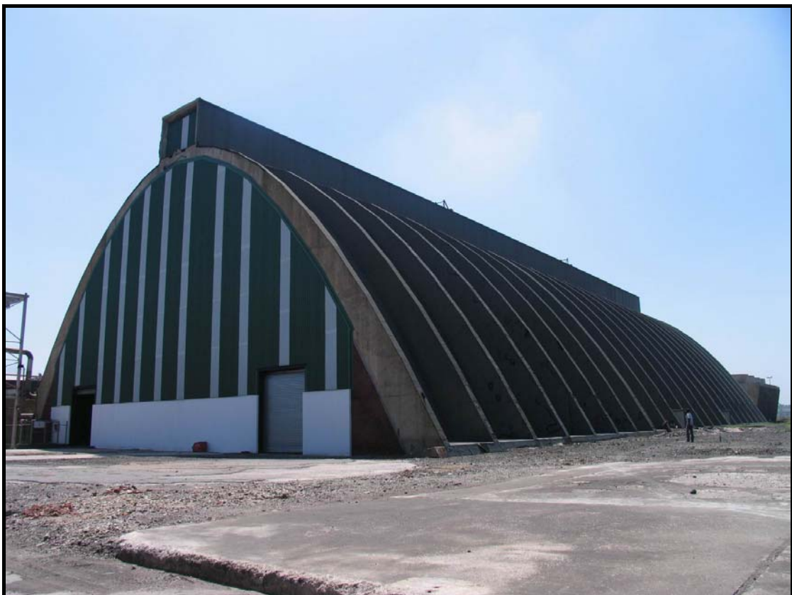
Figure 9. A purpose developed building from concrete
