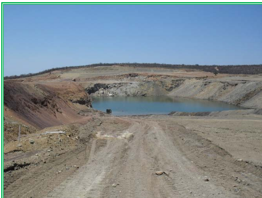
Fig 30: Opencast mining at Vele poses a threat to archaeological sites on the Colliery properties
