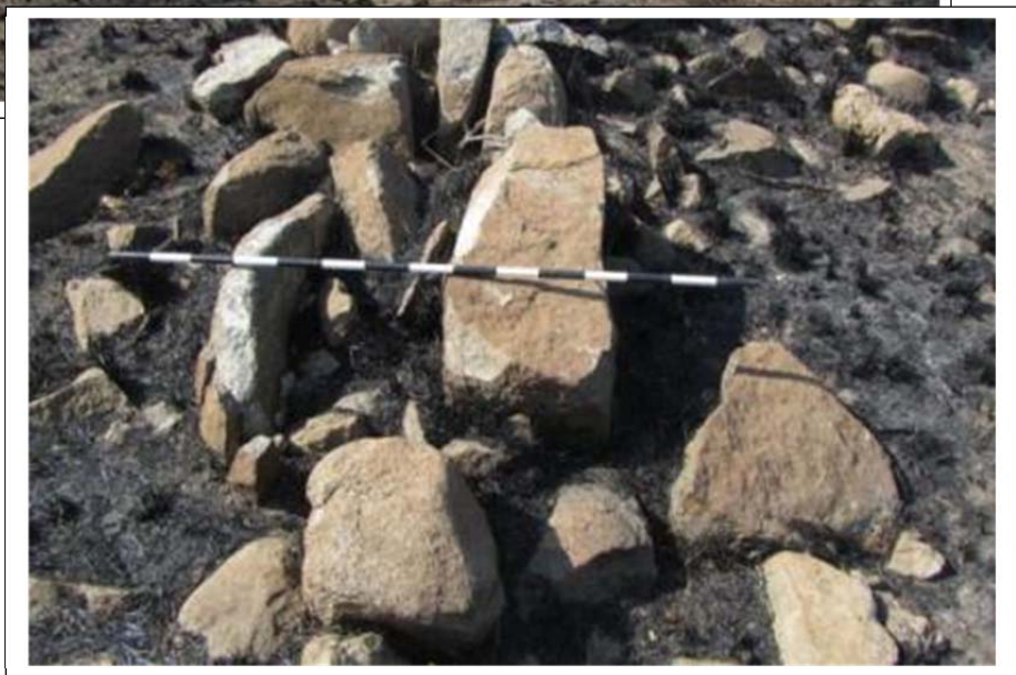
Figure 47- Cross section of Structure 07's wall indicates two parallel constructed lines of stone with rubble infilling. (Scale in 10cm intervals) (below).
