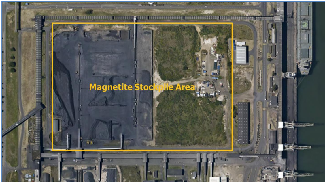
Figure 3-8: Existing Magnetite Stockpile Area
