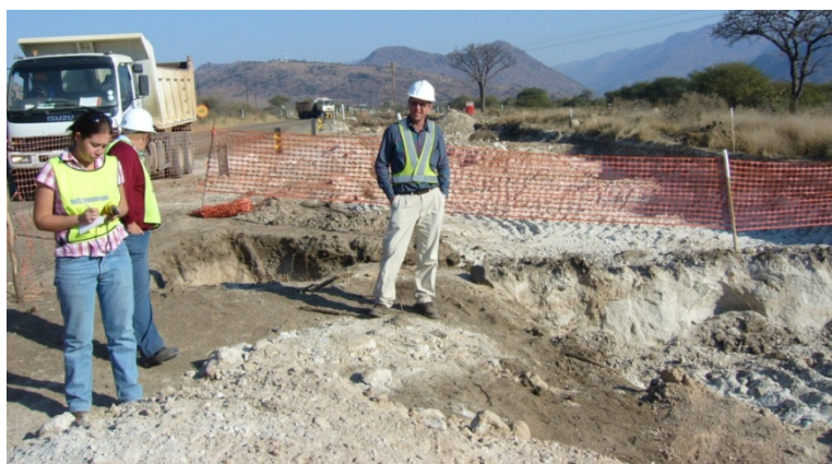
Figure 2. The excavation of the new Richmond road by the construction team, right next to the existing road. The skeletal remains were dislodged by the mechanical equipment.
