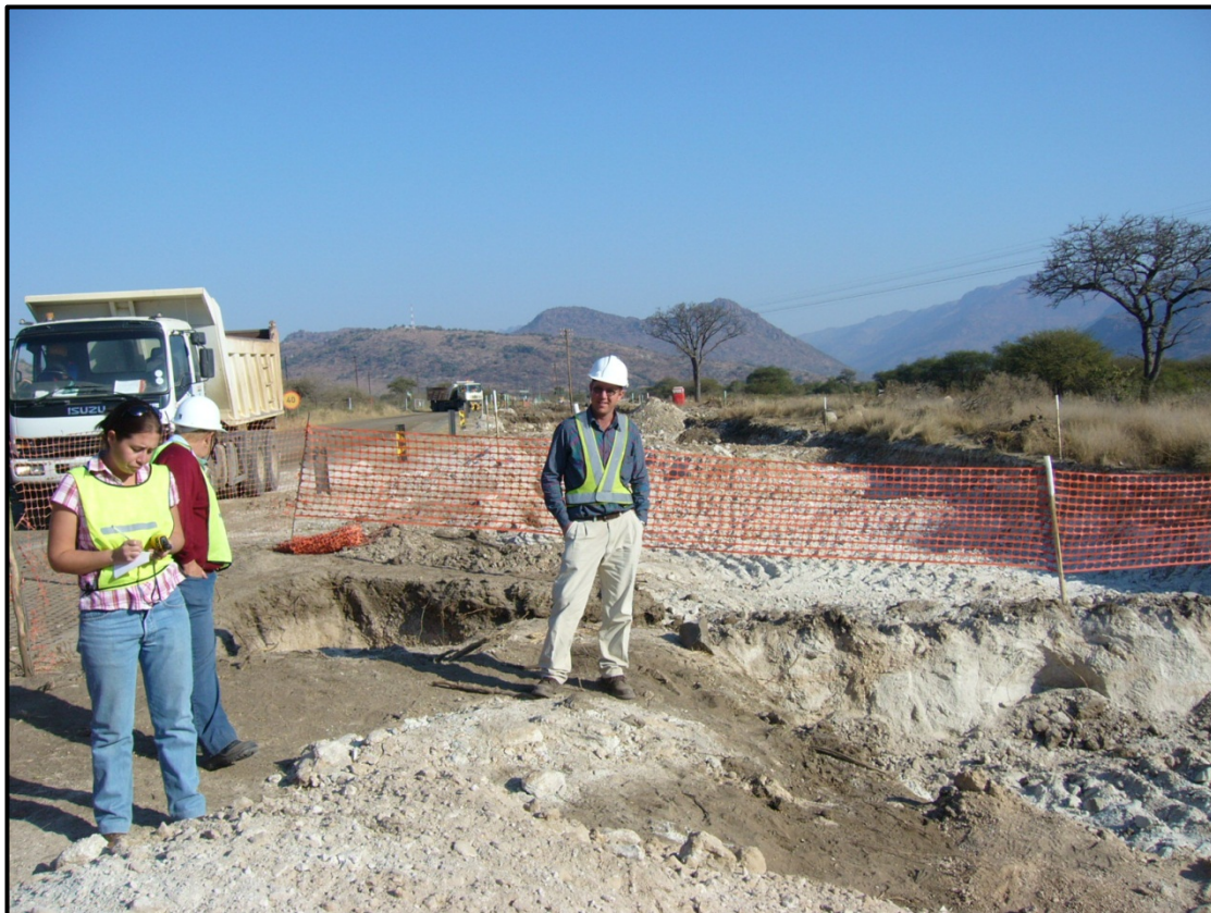
Figure 1. General view of the road construction area.
