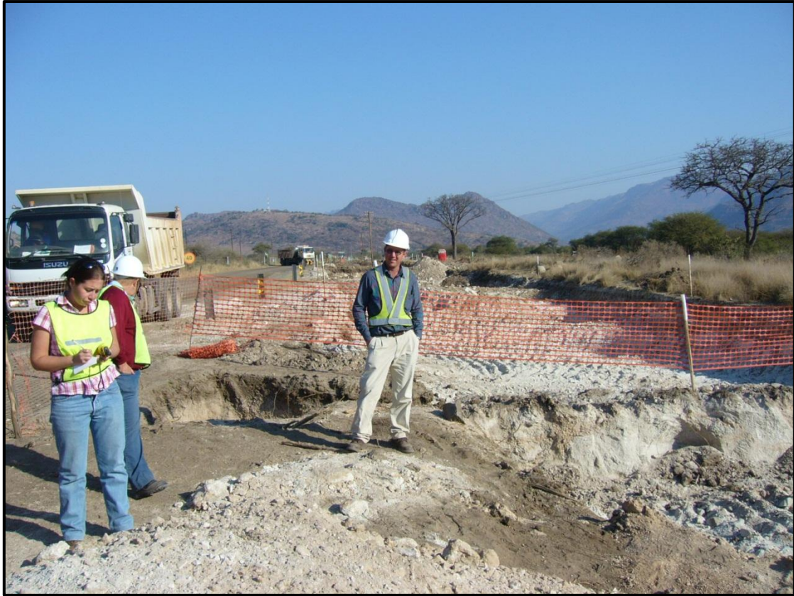
Figure 1. General view of the road construction area.
