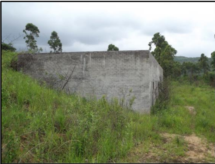
Figure 21: Structure 6 in a western direction.
