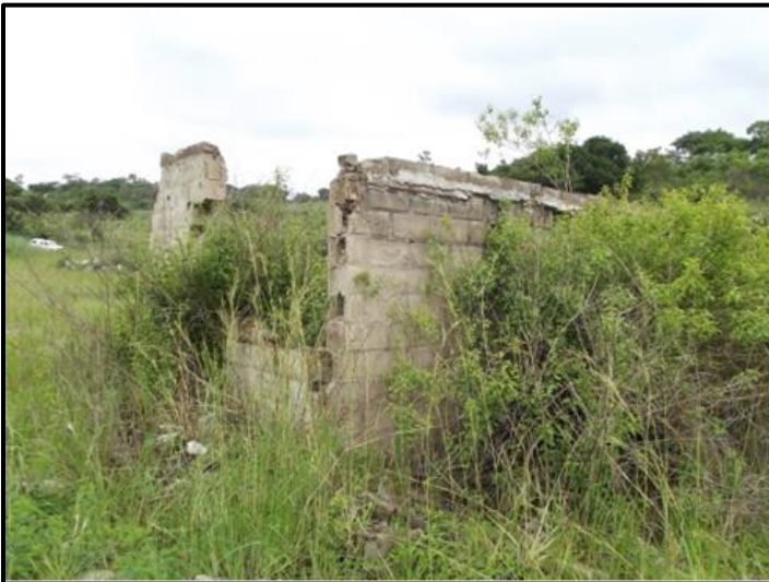
Figure 17: Structure 4 viewed from the North.
