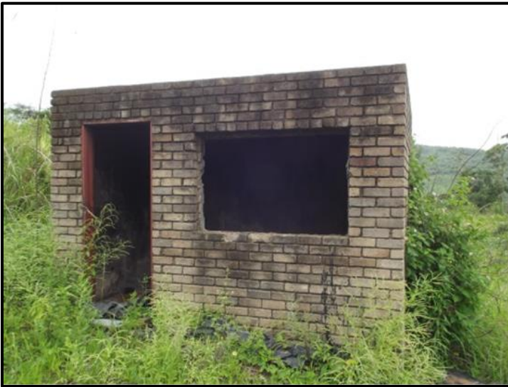
Figure 15: Structure 3 viewed in a northerly direction
