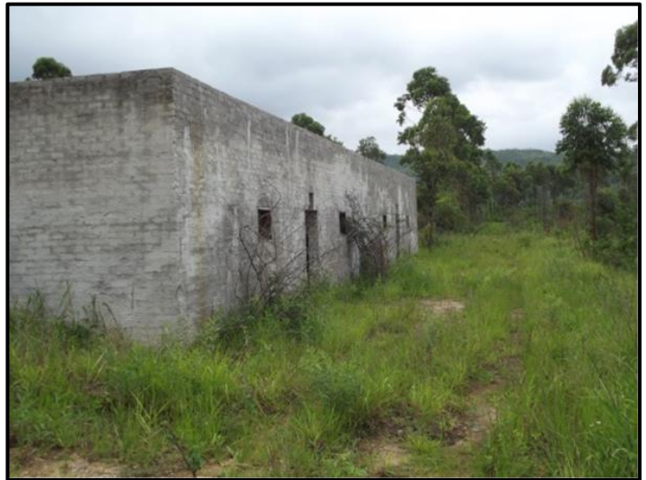
Figure 22: General view of structure 6.
