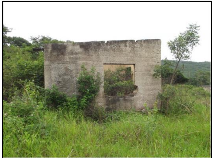
Figure 12: Structure 1 viewed from the West
