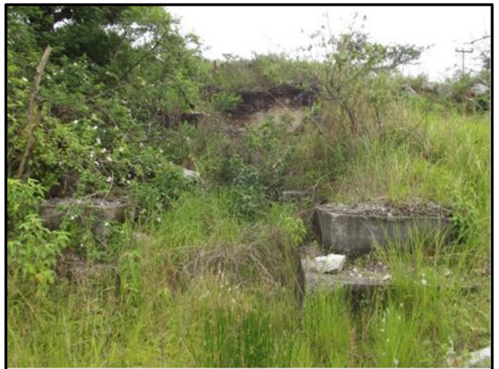
Figure 14: Structure 2 viewed in a westerly direction
