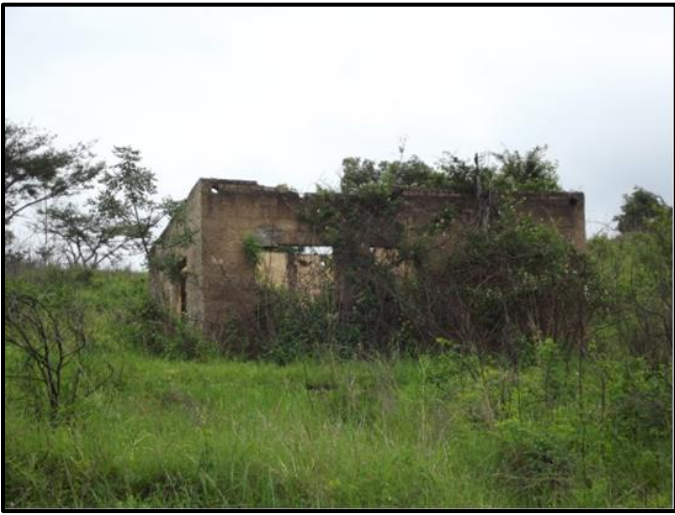
Figure 11: Structure 1 viewed from the North.
