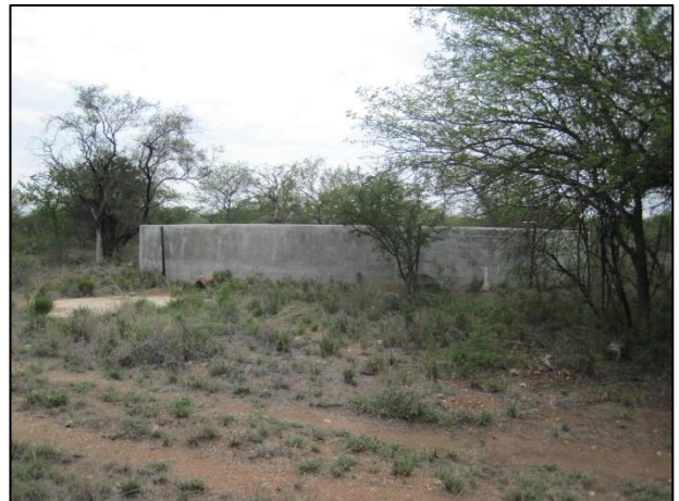
Figure 4: View of the large cement dam within the study area.
