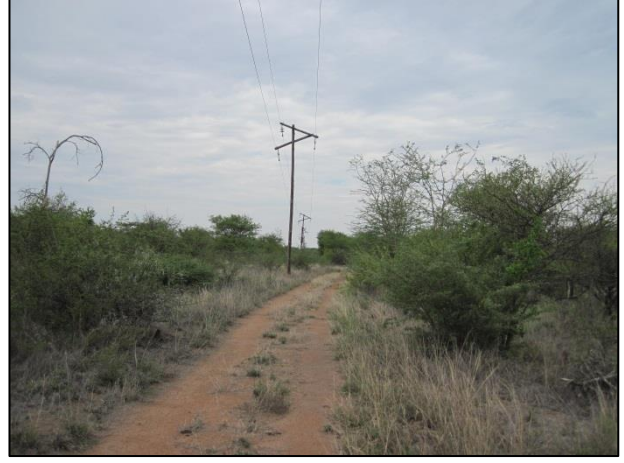
Figure 6: View of the power line adjacent and on the southern side of the study area.
