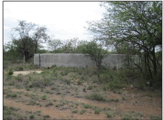
Figure 14: View of the large cement dam within the study area.
