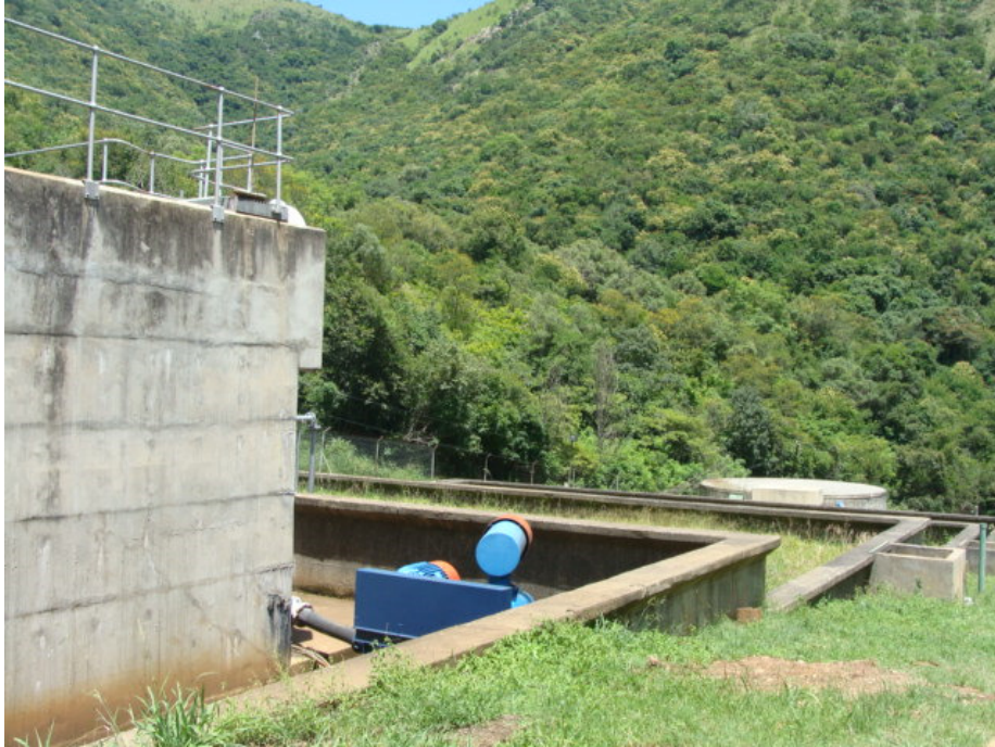
Figure 10: Existing WTW at Rimer's Creek.
