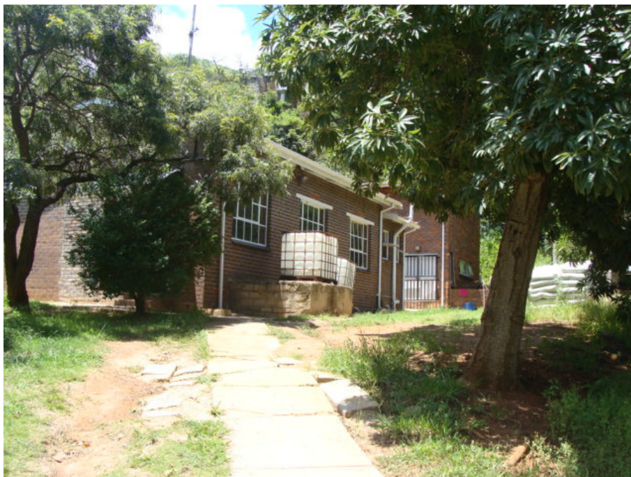
Figure 9: A building and other infrastructure at the existing WTW.
