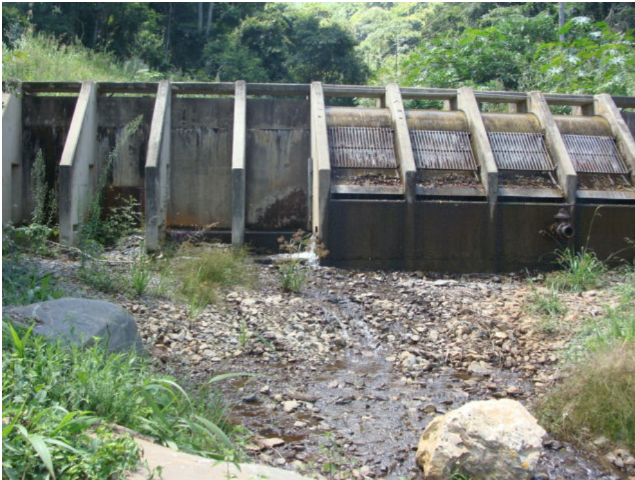
Figure 11: The existing weir at the WTW.
