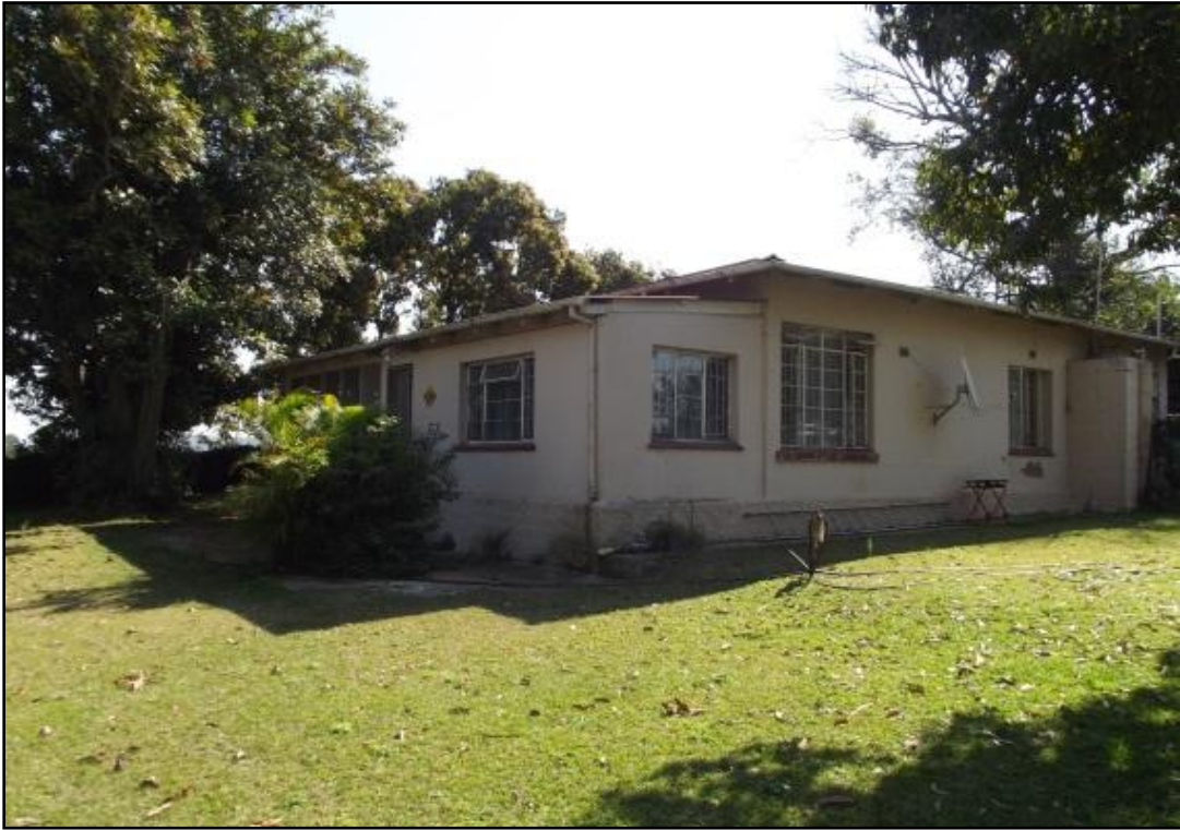
Fig. 1. Site NTC 1. An historic house. Eastern view.
