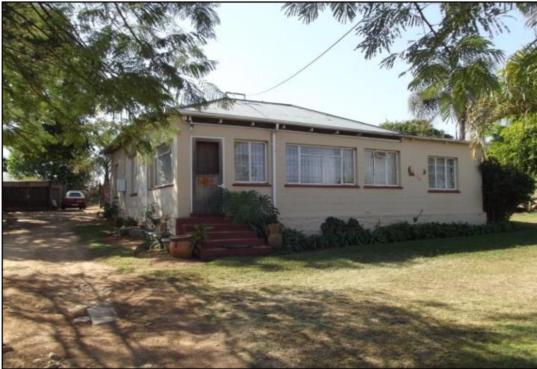
Fig. 8. Site NTC 5. View of the last historic house's southern face.
