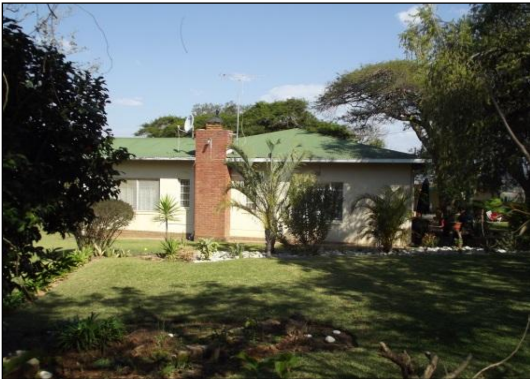
Fig. 4. Site NTC 2. Northern face of the second house.
