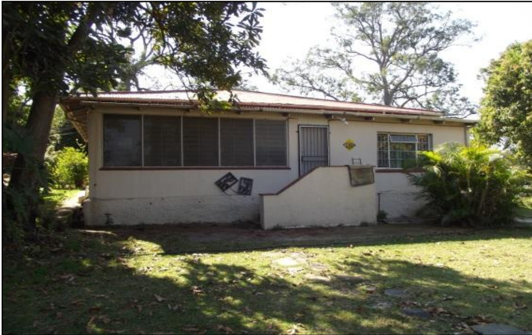
Fig. 2. Site NTC 1. The southern face of the house.
