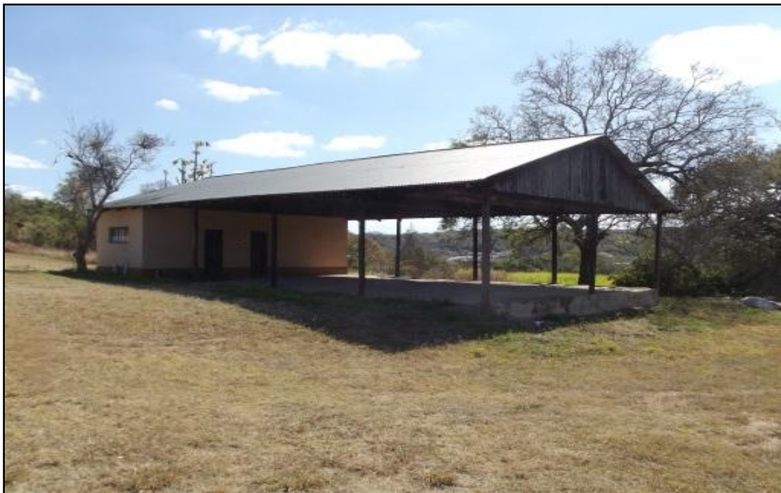
Fig. 18. Site NTN 11. A farm shed.
