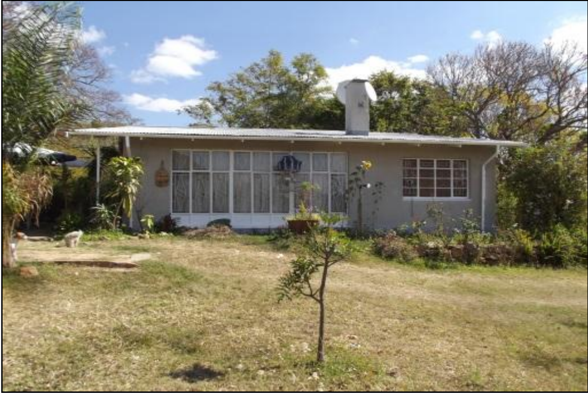
Fig. 17. Site NTN 10. A farm house which probably has historic significance as it is visible on old aerial photos.
