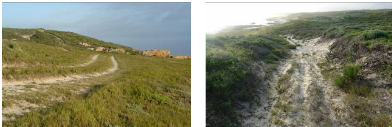
Fig. 33. View of the old eroded tracks.
