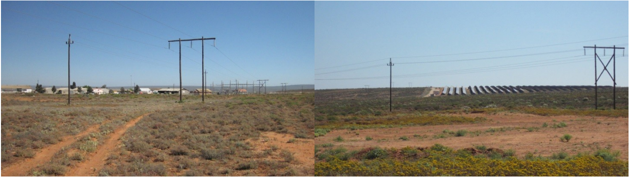
Plate 21: The existing powerline and Bulte sub-station on the edge of Vredenburg north. Plate 22: The existing PV facility to the north of Vredendal wich lies ~600 m to the nw of the Bulte sub-station
