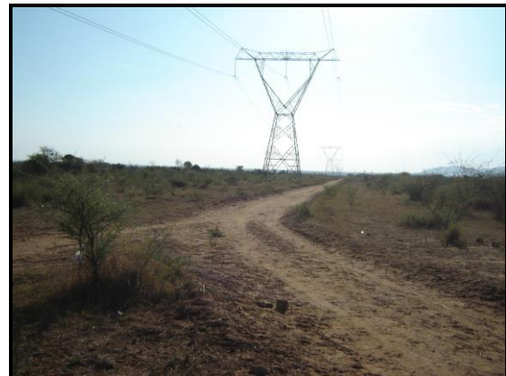
Figure 8: View of Access Road.
