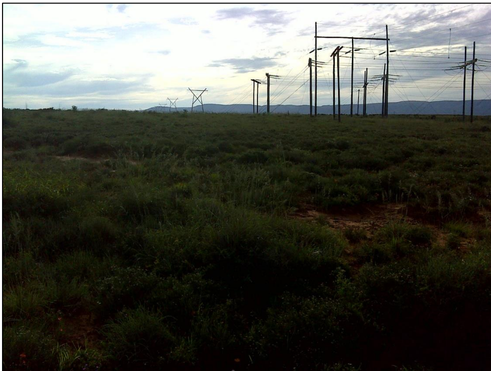
Figure 12. View of the area proposed for power line Alternative Path 2 from the Skilpad Substation showing the existing power line running parallel to the R75.
