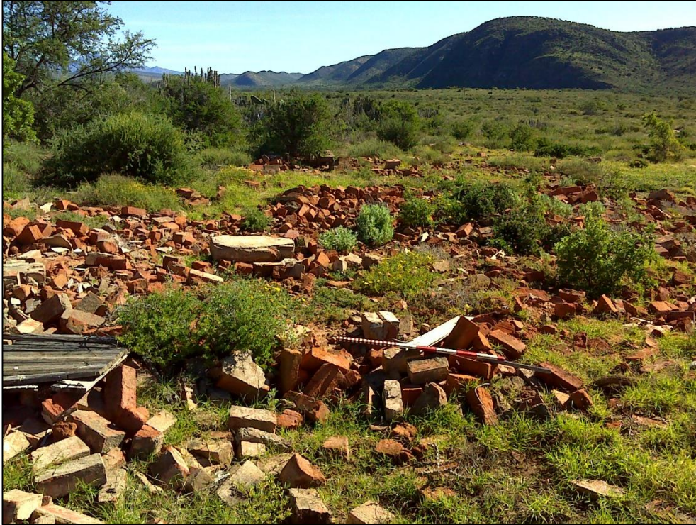
Figure 49. View of a dwellings' ruins situated within the area proposed for the development of infrastructure associated with the WEF project on the Farm Adolphs Kraal.
