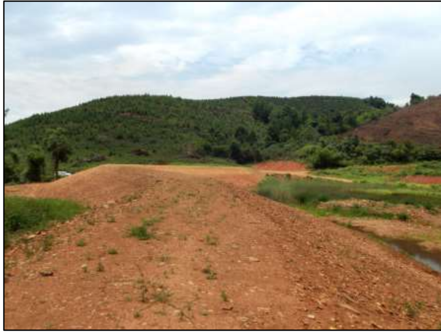
Figure 6. Site SO 4. Photo taken in a south-eastern direction.
