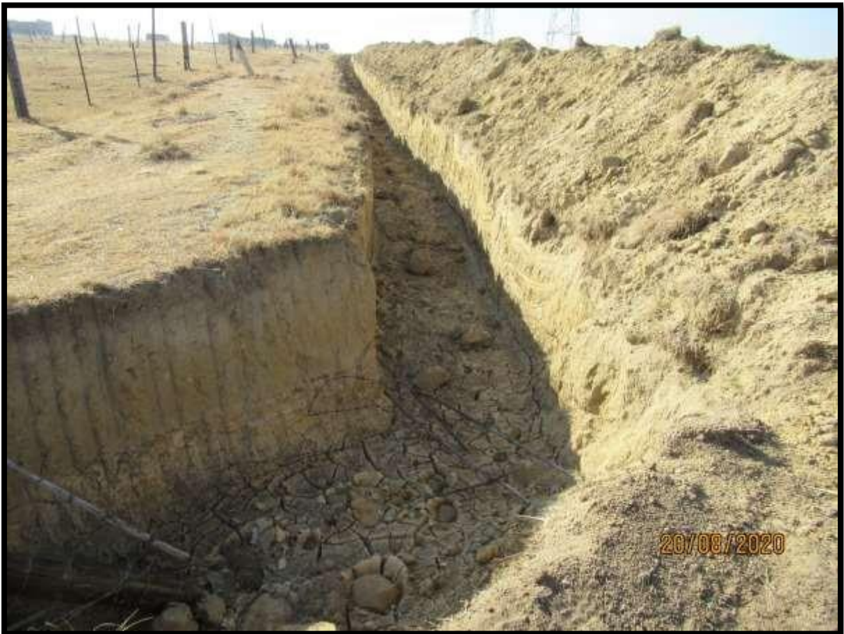
Figure 12: Channel showing depth of overburden.
